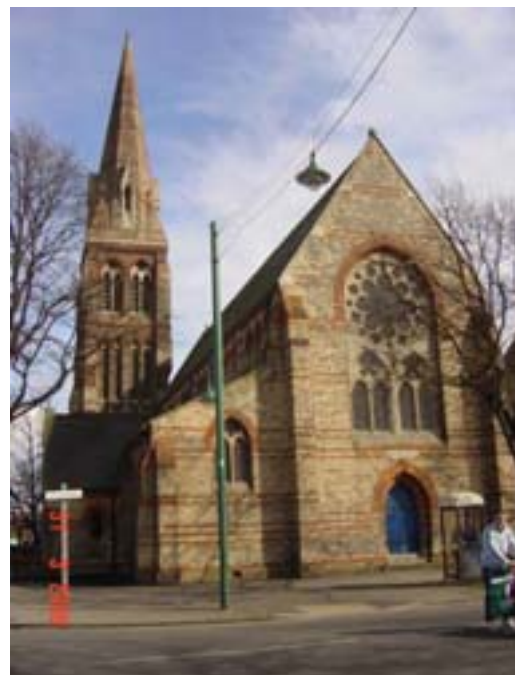
fig 18 St. Matthew's Church [Listed Grade 2]
