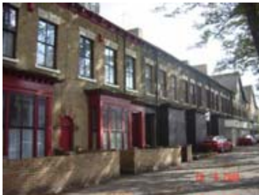
fig 2 Nos 247-253 boarded up frontages.
