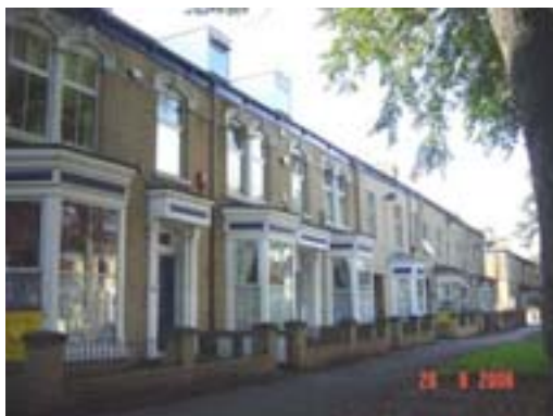
fig 16 Nos 98-102, dwarf walls with railings.
