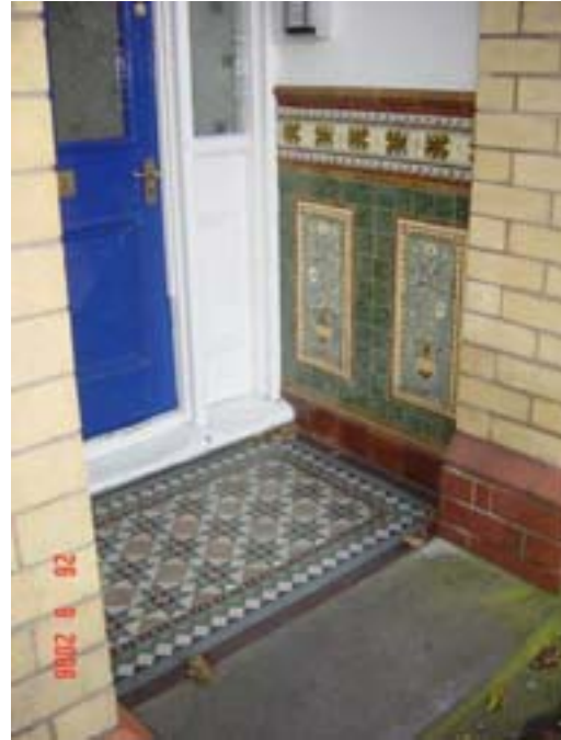
fig 4 No 163 Decorative tiled porches are a feature of the Conservation Area.
