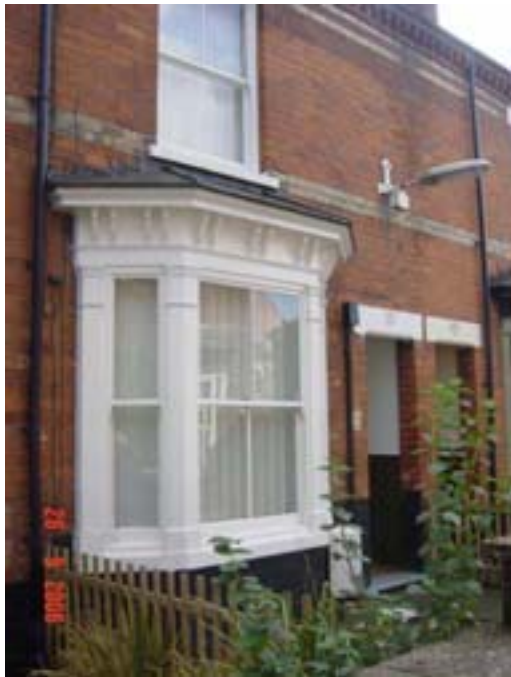
fig 8 Original windows, Albert Avenue
