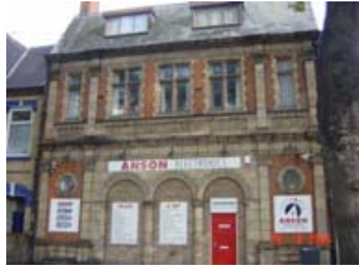
fig 10 Former Western Hull and Sculcoates Dispensary.
