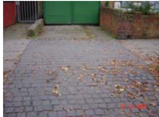
fig 25 Two types of setts in vehicle crossing.
