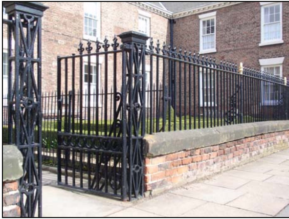
Photo 13: Iron gate, piers and railings in front of the Charterhouse.
