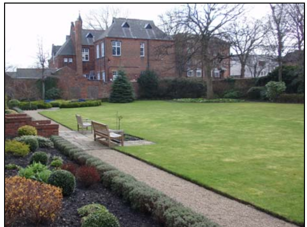
Photo 26: The old main school block from the Master's garden.
