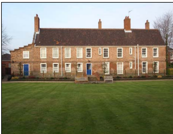
Photo 15: The rear elevation of the Master's House.
