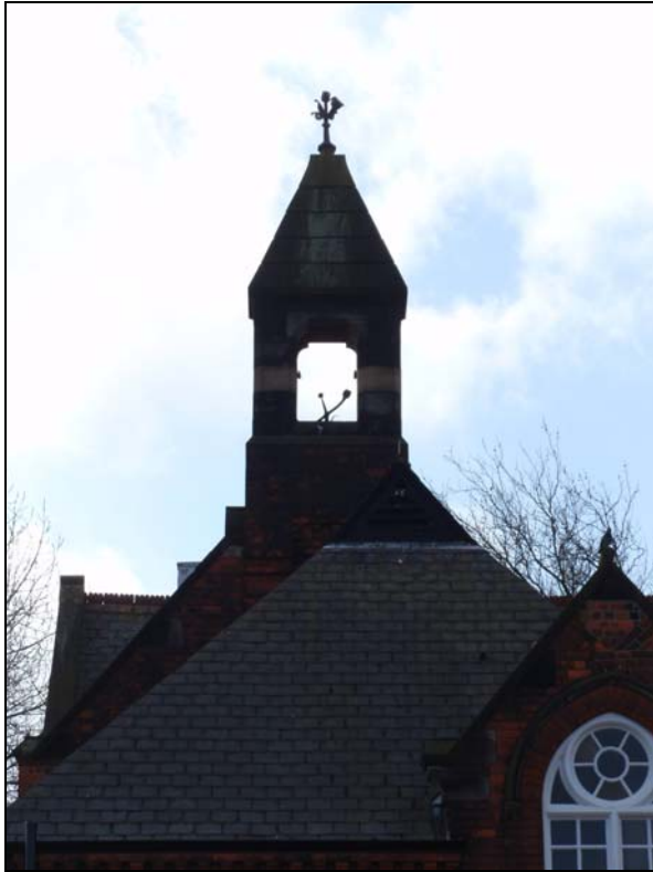
Photo 23: Bellcote on the old Charterhouse Lane school (main block).
