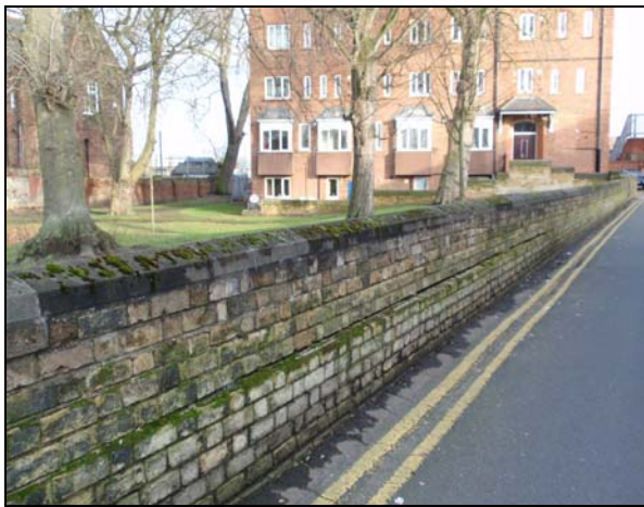
Photo 29: Boundary wall (outer south face), old Burial Ground.
