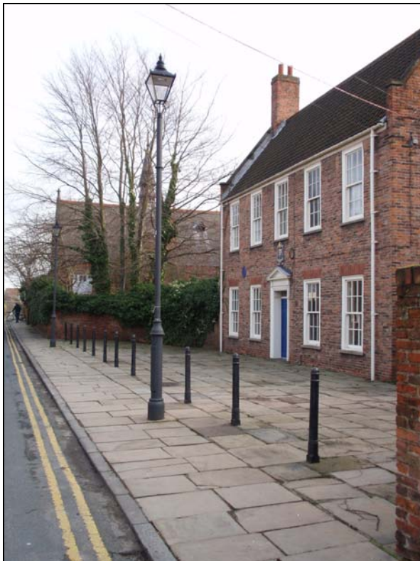
Photo 20: Forecourt to the front of the Master's House, Charterhouse Lane.
