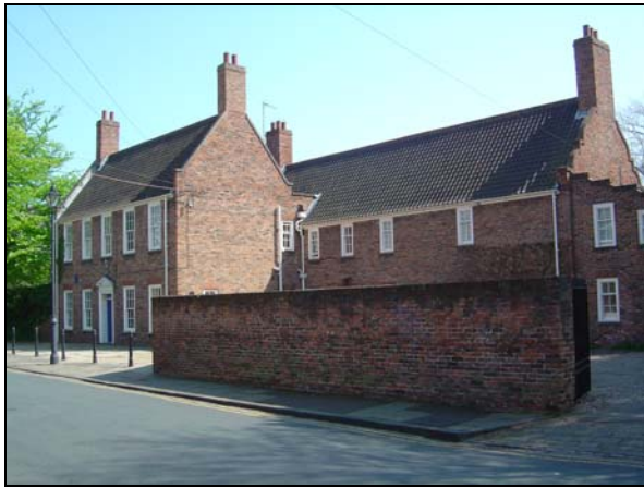
Photo 14: The Master's House, Charterhouse Lane.
