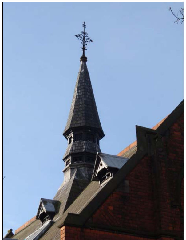
Photo 22: Ornate octagonal bell turret on the old Charterhouse Lane school (infants' block).
