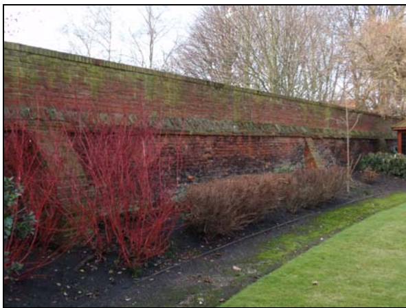
Photo 8: Boundary wall on the west side of the Master's garden.
