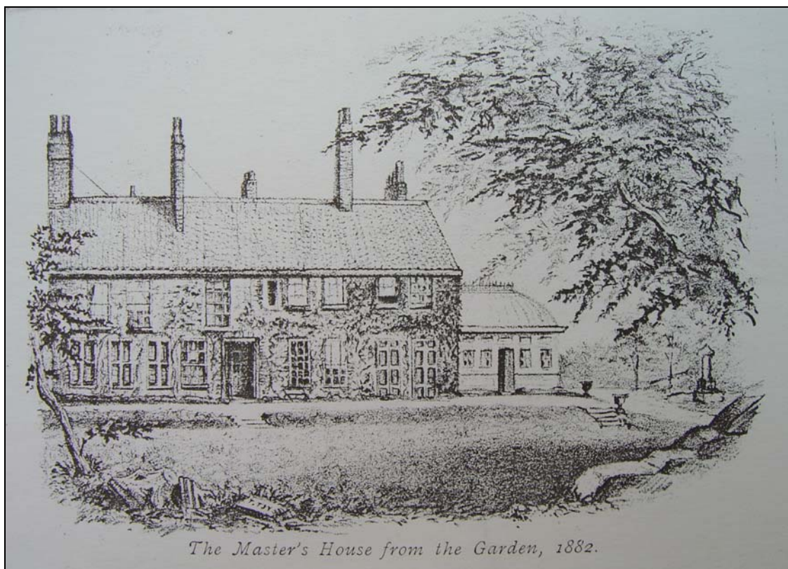
Figure 16: The Master's House from the Garden in 1882 (illustrated in Cook's 'History of God's House of Hull', 1882). To the right of the Master's House there is an orangery; to the far right what appears to be a stone cross (also evident in Figure 15); and in the foreground (bottom left) some architectural fragments, including a capital, possibly from the old priory.
