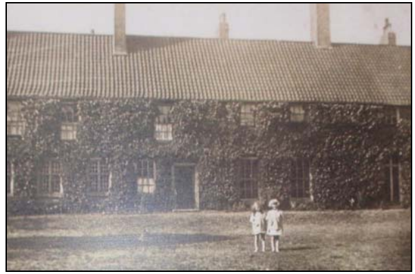
Photo 16: The rear of the Master's House, c.1920s with the stone cross-windows in evidence on the ground floor (left hand side) (courtesy of the Master of the Charterhouse).
