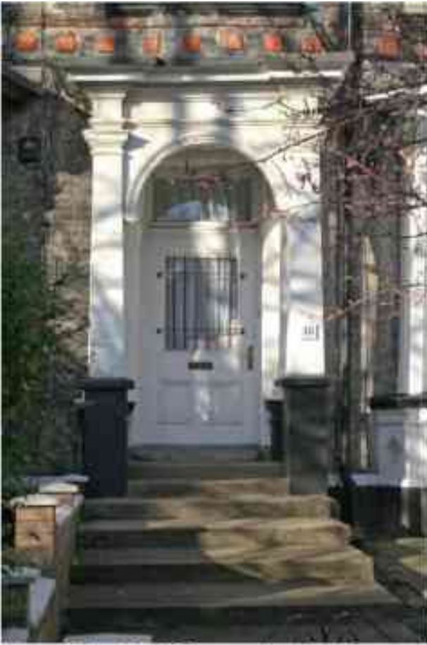
Figure 175 No.10 Pearson Ave front door
