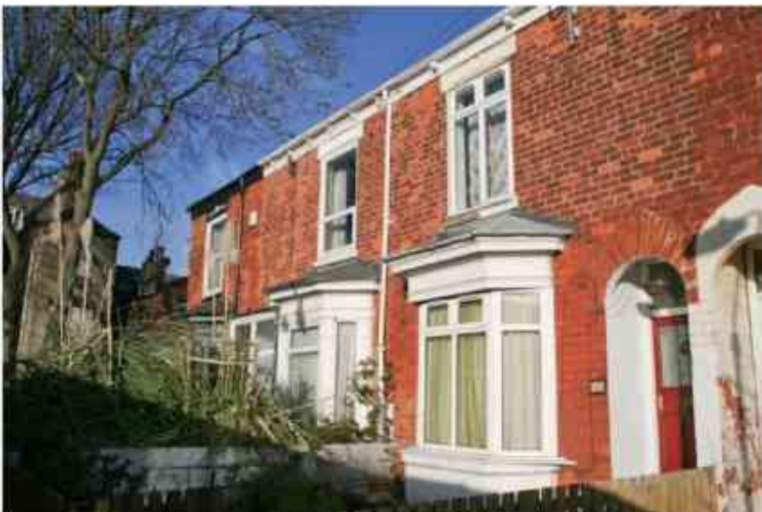
Figure 205 West View Nos. 8 to 6
