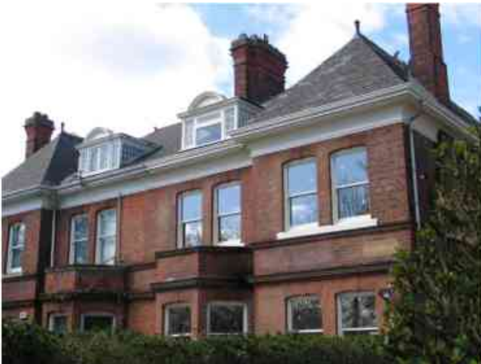
Figure 114 No. 49 angle with replacement double-glazed timber sash windows
