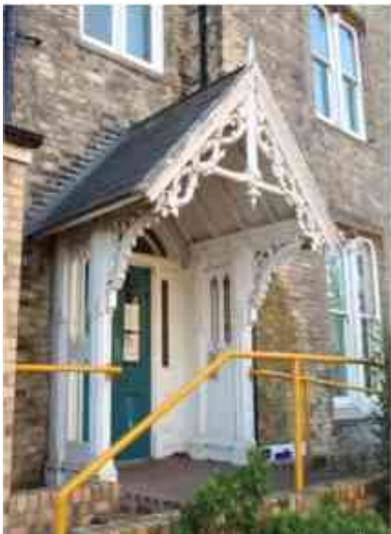
Figure 63 Police Station – side entrance detail
