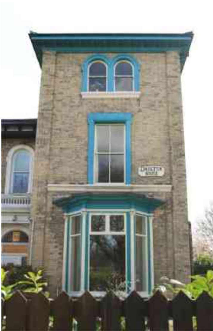
Figure 66 No. 20a Daulton House
