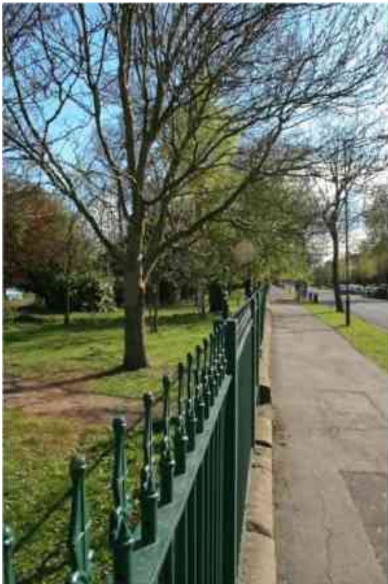
Figure 30 New railings showing Princes Avenue boundary
