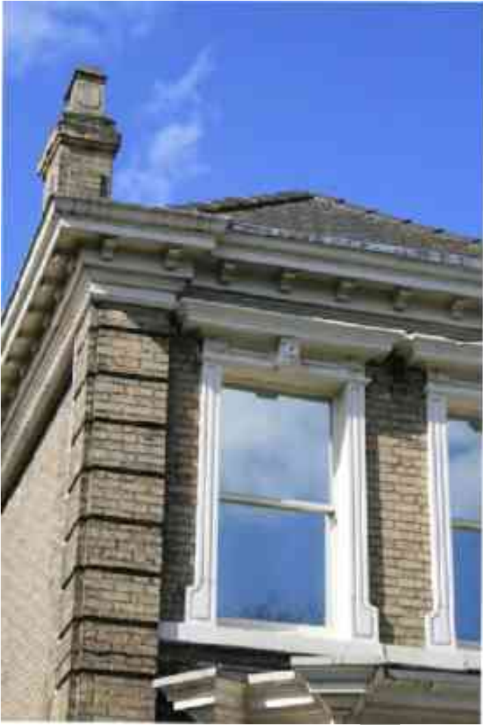
Figure 116 No. 50 first floor window and roof
