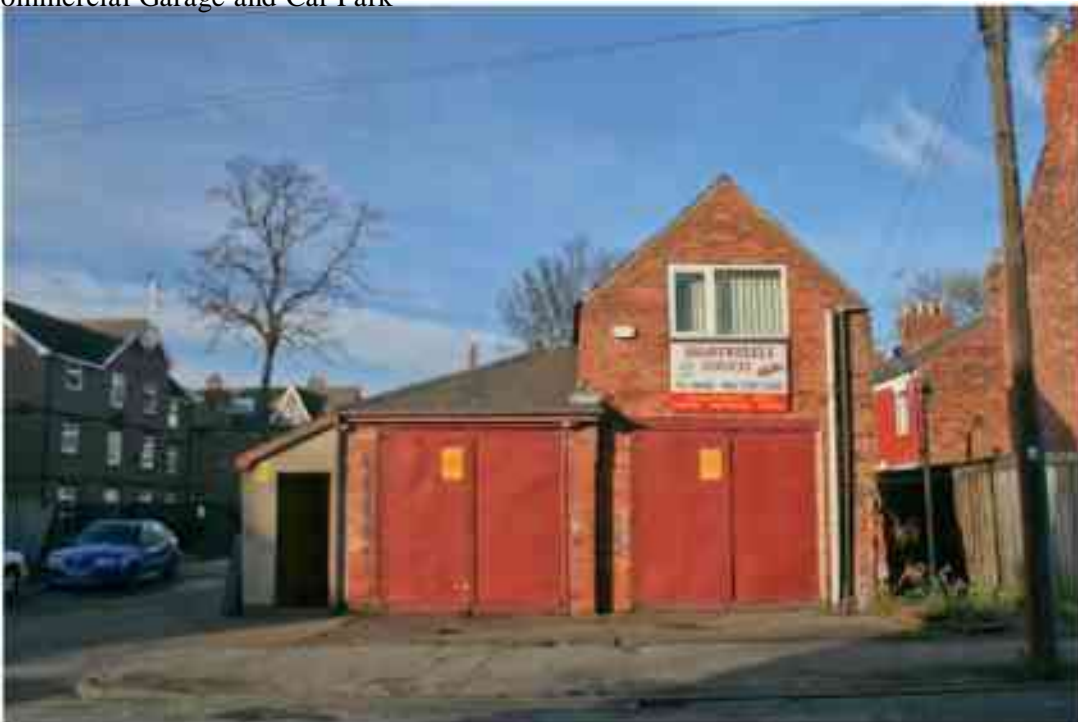
Figure 207 Commercial Garage front, Grove Street
