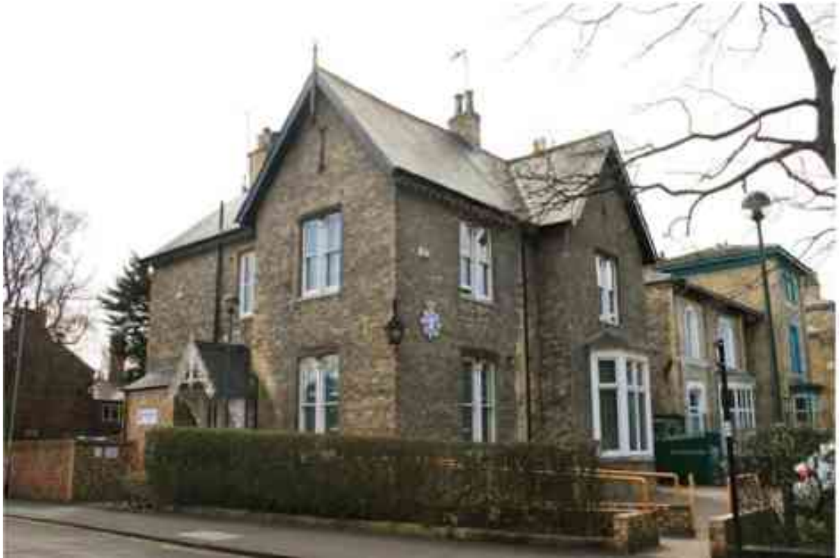
Figure 62 Police Station or Keysell Villa – diagonal
