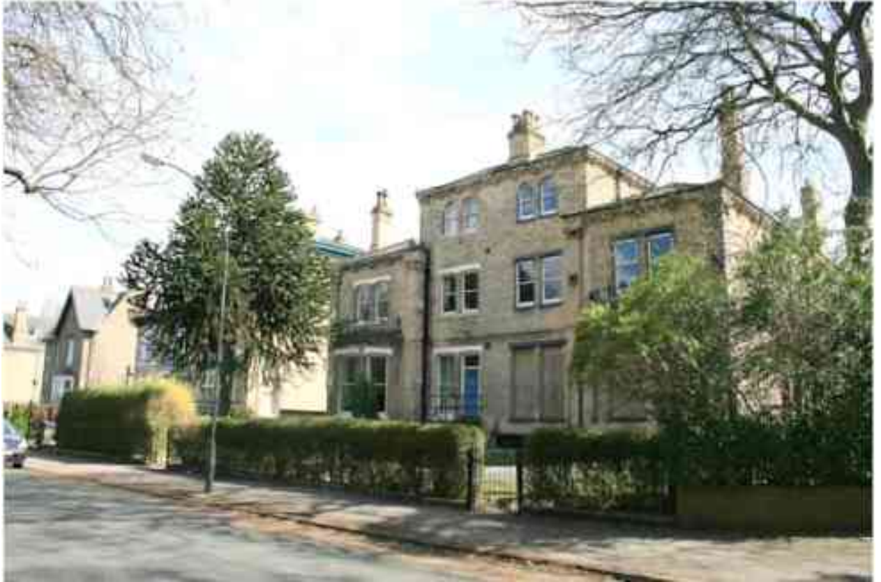
Figure 69 Nos. 21 & 22 street view
