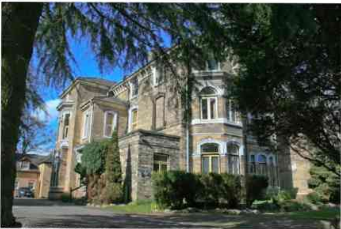
Figure 128 Side of No. 56 through trees
