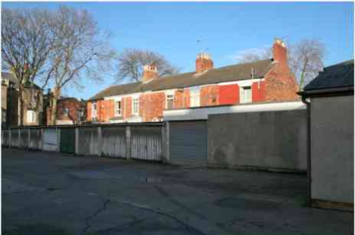
Figure 209 View of West View
