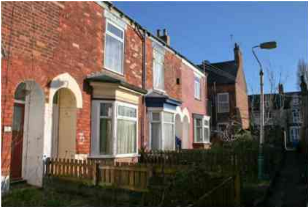
Figure 204 West View Nos. 4 to 1
