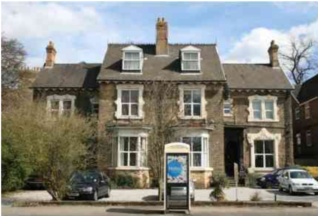
Figure 47 Nos. 2 & 3, or Leicester Cottage , front view
