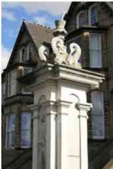
Figure 11 Pearson Park Gate pillar detail
