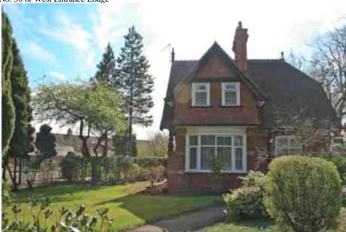
Figure 84 West Lodge and garden
