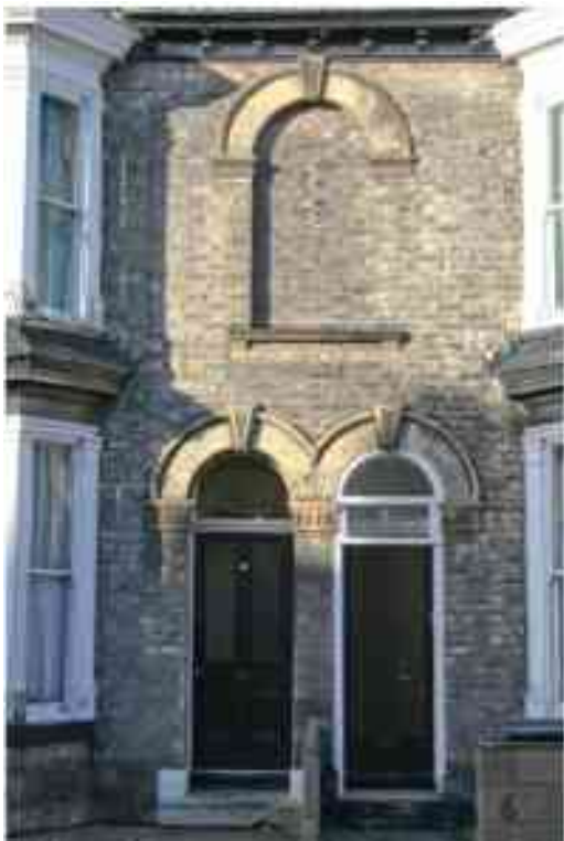
Figure 200 Nos. 6 & 8, Grove Street, front doors
