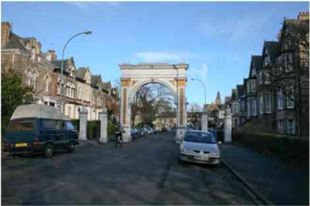
Figure 190 Pearson Avenue view of gateway from inside park
