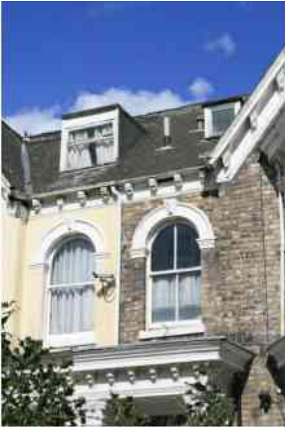
Figure 158 Nos. 72 & 74 arched window detail
