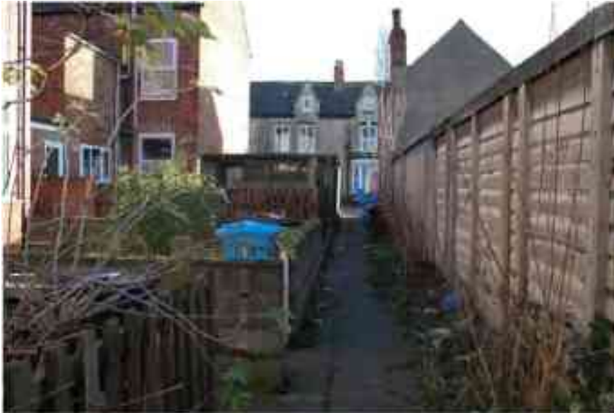
Figure 206 View of Grove Street from West View
