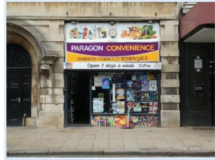
Figure 55 Out of proportion fascia advertisement at Grade II 88 & 90 Paragon Street
