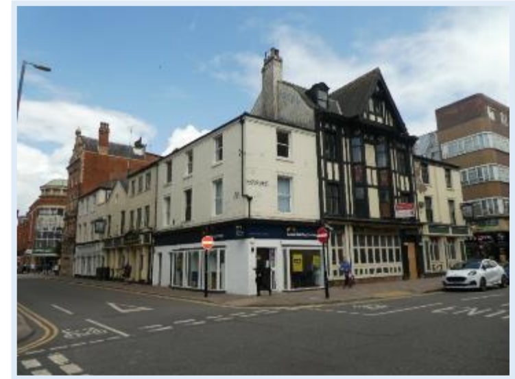
Figure 16 Paragon Street & South Street
