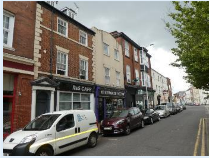
Figure 82 Key and Positive Buildings along Story Street
