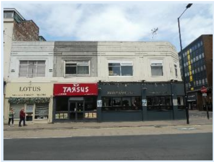
Figure 50 Lack of Uniformity at Queen Street
