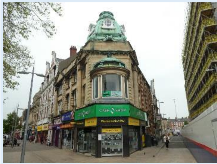
Figure 22 Grade II 46, 48 & 50 King Edward Street
