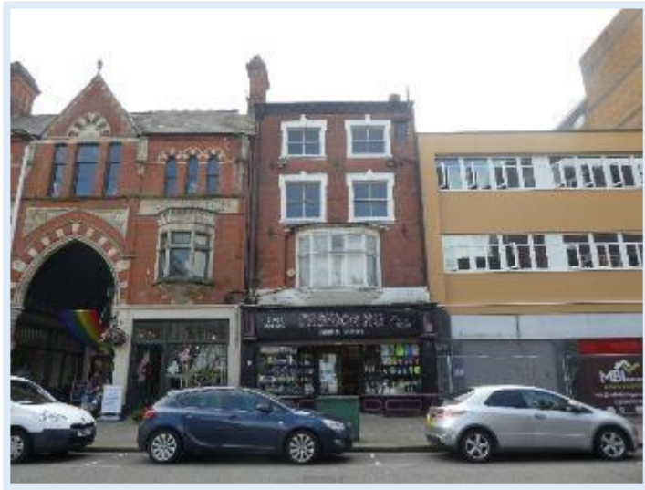
Figure 63 Historic Sash windows 55 Paragon Street
