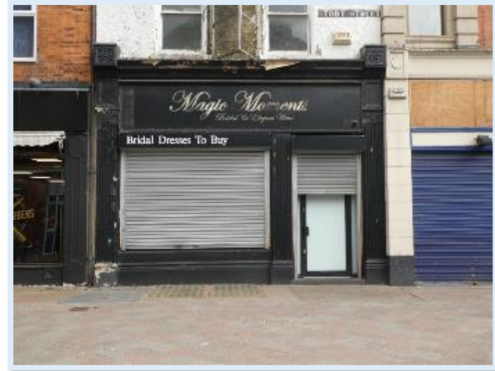
Figure 45 Remnants of a .19 th Century shop front at 14 Story Street
