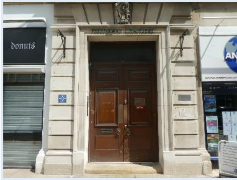
Figure 66 Original Door at Ferensway Chambers
