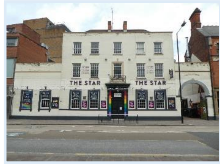
Figure 60 - Georgian Revival Inn on Carr Lane
