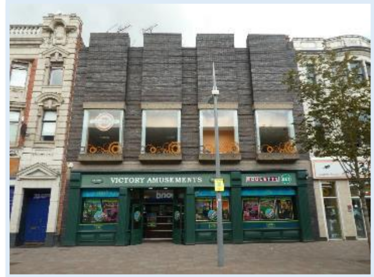
Figure 36 Modernism on King Edward Street
