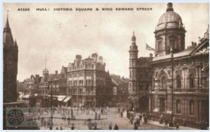
Figure 6 Lost Edwardian Hull (East Riding Archives) – site of Triangle Building
