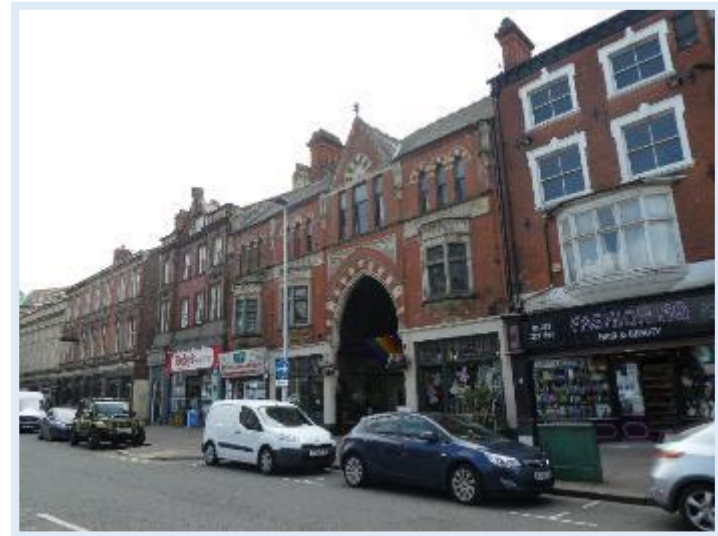
Figure 85 Key and Positive Buildings along Paragon Street
