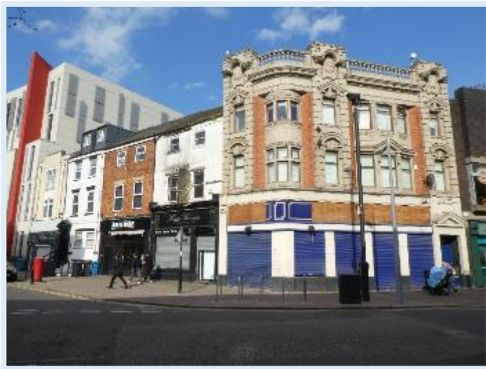
Figure 83 Positive Buildings at Story Street and King Edward Street
