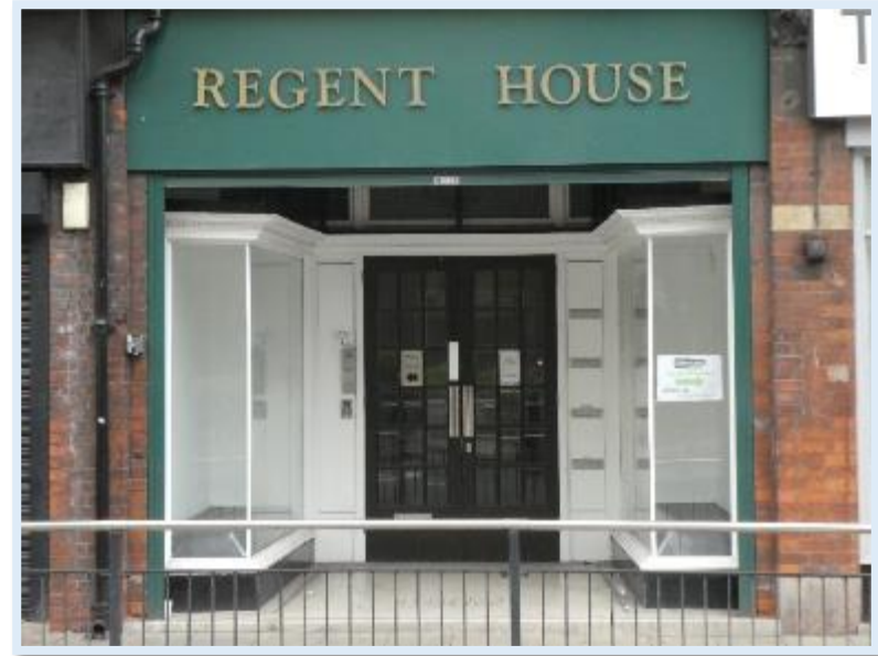
Figure 38 183 Ferensway – The best preserved original shop front within the Conservation Area.
