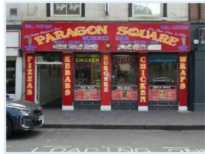
Figure 56 'Cluttered' Shop front at 14 Paragon Square
