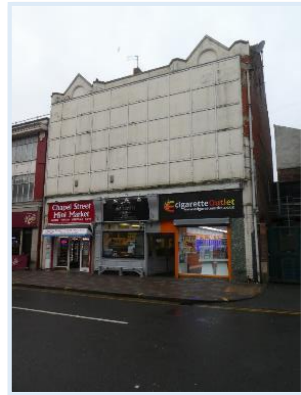
Figure 86 Potential to restore the 19th century frontage of the 'Archeron shop', Chapel Street.
