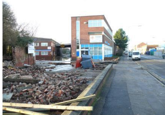
Wall destroyed by flood waters, English Street
