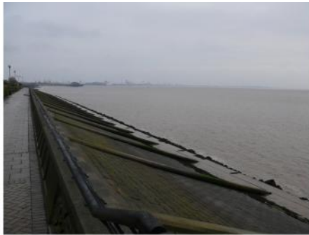
Victoria Dock, showing riverside defence wall at low tide (left) and evidence of over-topping (right).
