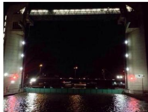
Hull Tidal Surge Barrier in operation, 5 th December 2013
