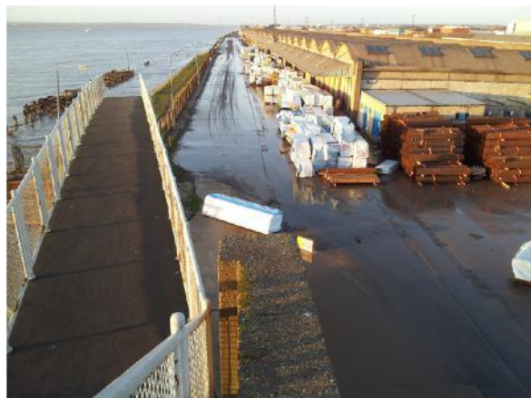
Hull Humber frontage defences
