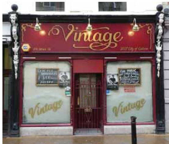
Existing traditional shop fronts
