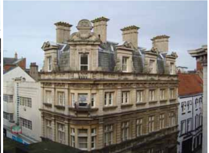
Former Britannia Building Society, 67 Whitefriargate
