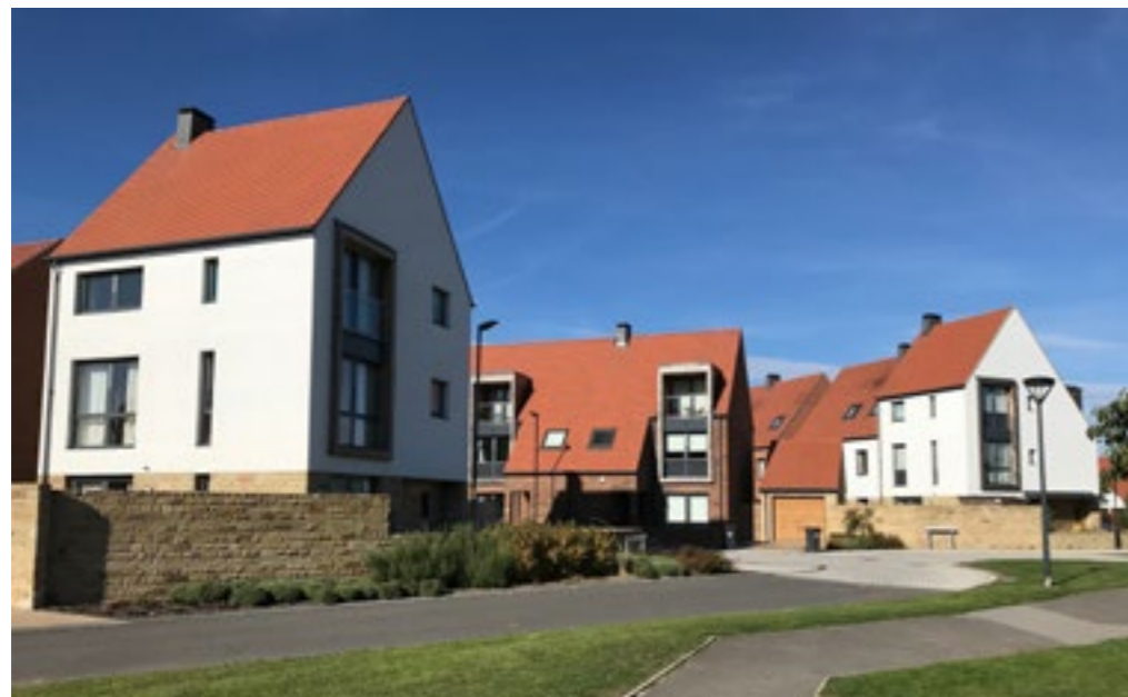
Fig 15: Derwenthorpe, York - bespoke corner turning house designs provide surveillance of the public realm and make a feature of the corner plot houses
