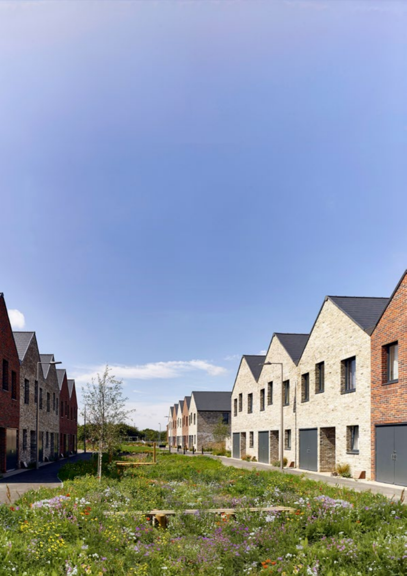
Fig 29: St. Chad's, Thurrock. Cars are excluded from the central street and the swale is made the focus for the main pedestrian route through the site.
