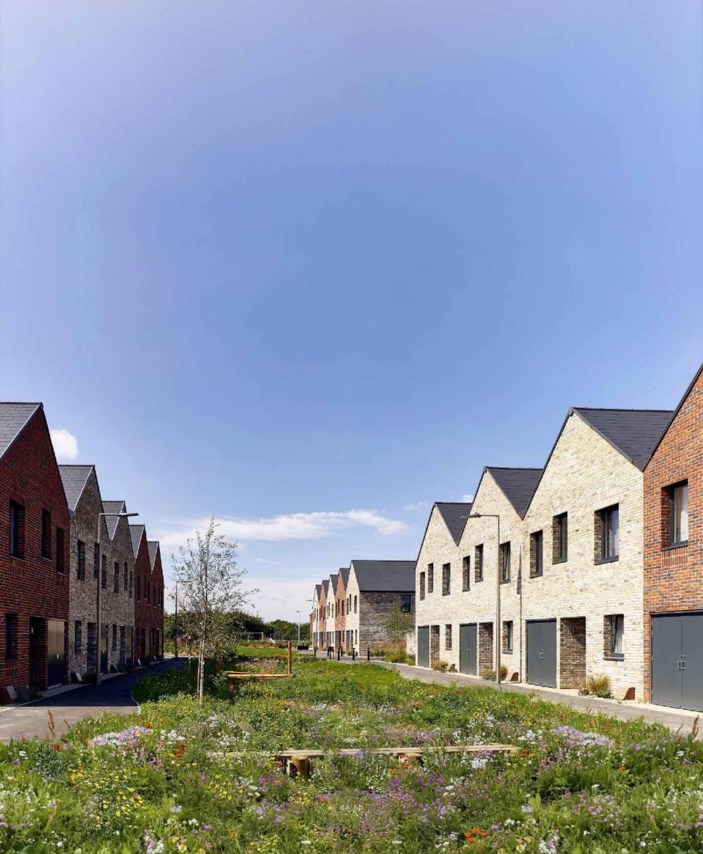
Fig 19: Example of a 'SUD Street' at St. Chad's, Thurrock. Cars are excluded from the street and the swale is made the focus for the main pedestrian route.
