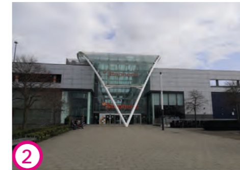
2 Pedestrianised area outside St Stephen's shopping Centre
