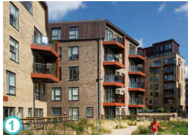
Example of medium density residential apartment buildings with 3 - 5 storeys
