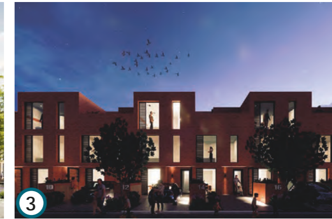
3 Langworthy Terraces: precedent showing the opportunity for a mix of housing types
