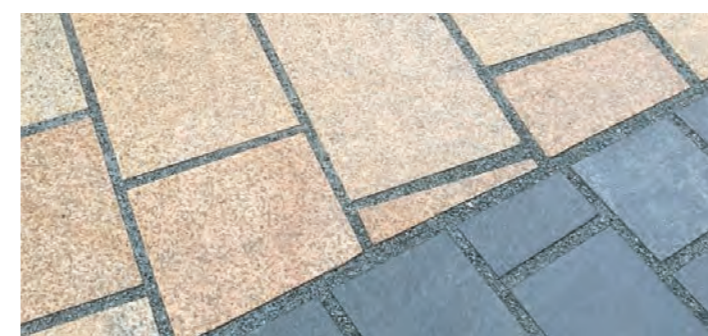
Figure 6.13: Example of Permeable Paving
