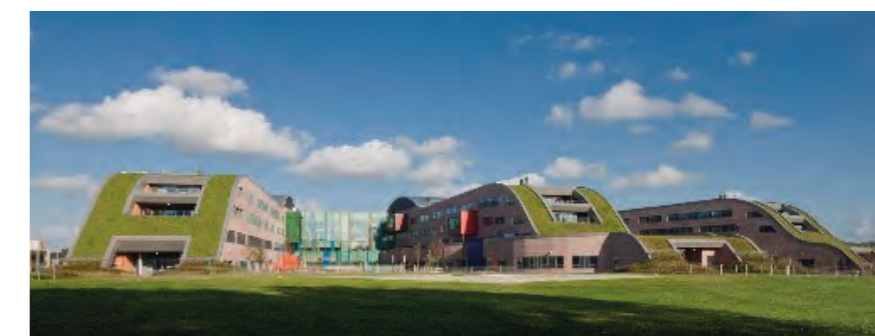
Figure 6.12: Example of Green Roof – Alder Hey Hospital
