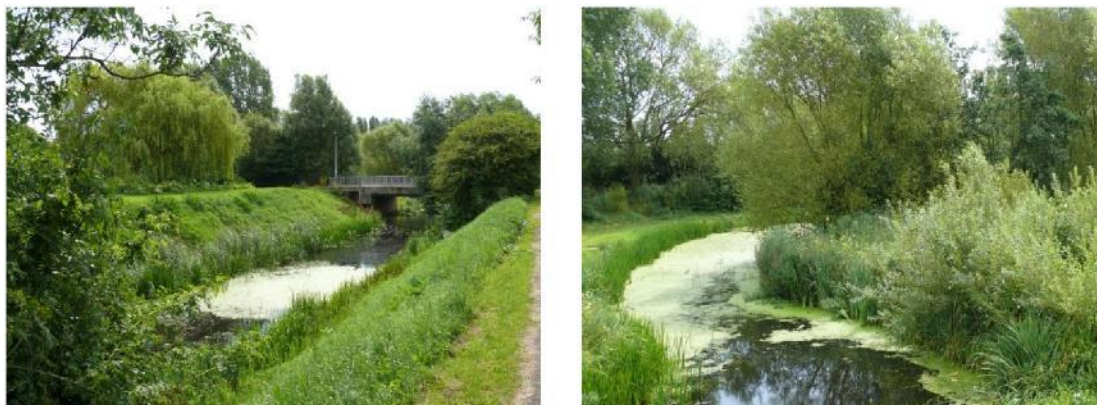
Beverley and Barmston Drain
