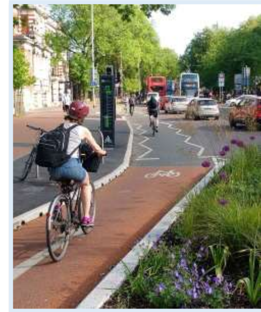
Figure 33 - Cycle routes in Manchester with landscape buffers between cyclists and vehicles (Wikipedia, 2023)
