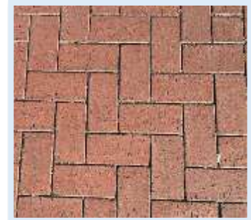
Figure 48 - Terracotta bricks on the approach to road junctions and to define retail frontage boundary (Author, 2023)
