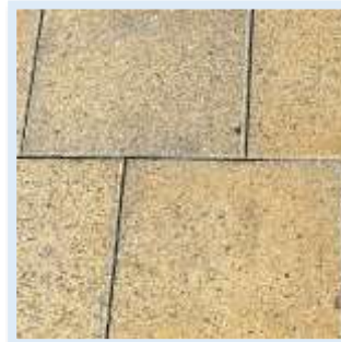
Figure 49- Buff paving slabs to general footpaths (Author, 2023)
