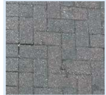
Figure 47 - Grey brick sets to define pedestrian crossing points to adjoining roads (Author, 2023)
