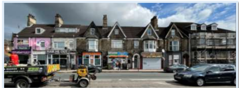
Figure 44 - Photograph of 230 to 246 Spring Bank (north) (Author, 2023)
