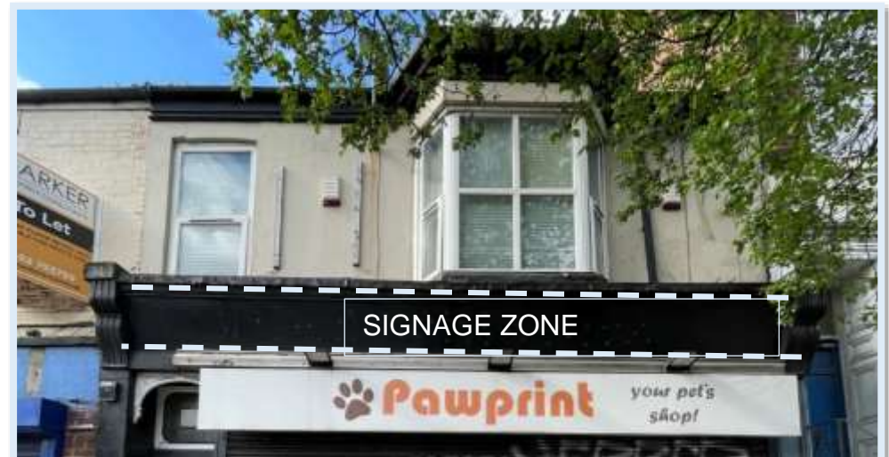
Figure 109 - 45 Spring Bank has retained its original fascia, cornice and corbels but the signage is positioned below the signage zone (Author, 2023)
