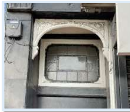
Figure 79 - Cast iron arched doorway detail and decorative fanlight retained (Author, 2023)
