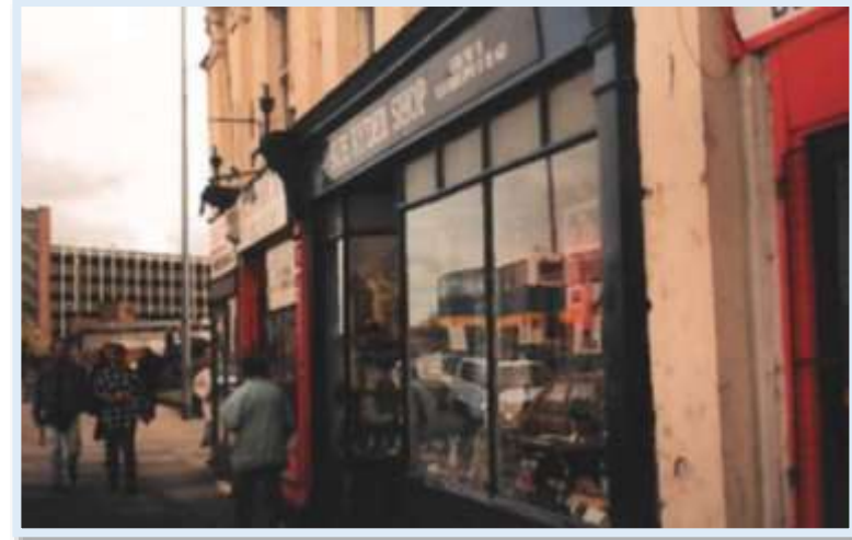
Figure 102 - 19 Spring Bank in 1995 shortly before Conservation Area Designation with the traditional shopfront retained including the recessed door and fanlights (Hampel, 1995)
