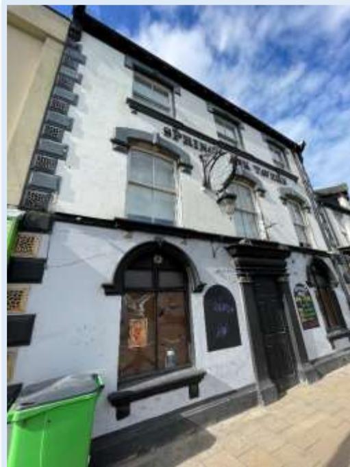
Figure 77 - Render utilised to the external walls of the Spring Bank Tavern (Author, 2023)
