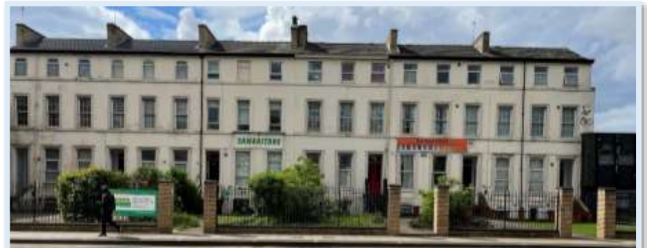
Figure 56 - Photograph towards 69-79 Spring Bank (south) (Author, 2023)
