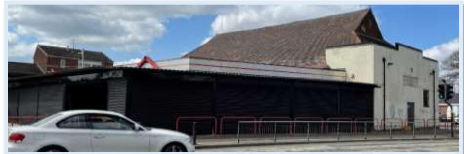
Figure 69 - No 185 Spring Bank which comprises of the former Church Hall to St Jude's Church and a later 1980's extension which fronts the adjacent car park, breaking the building line and massing (Author, 2023)
