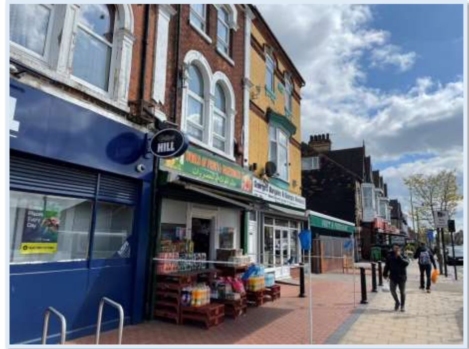
Figure 66 - Photograph of 186-188 Spring Bank showing the generous extent of external areas to some retail units (Author, 2023)
