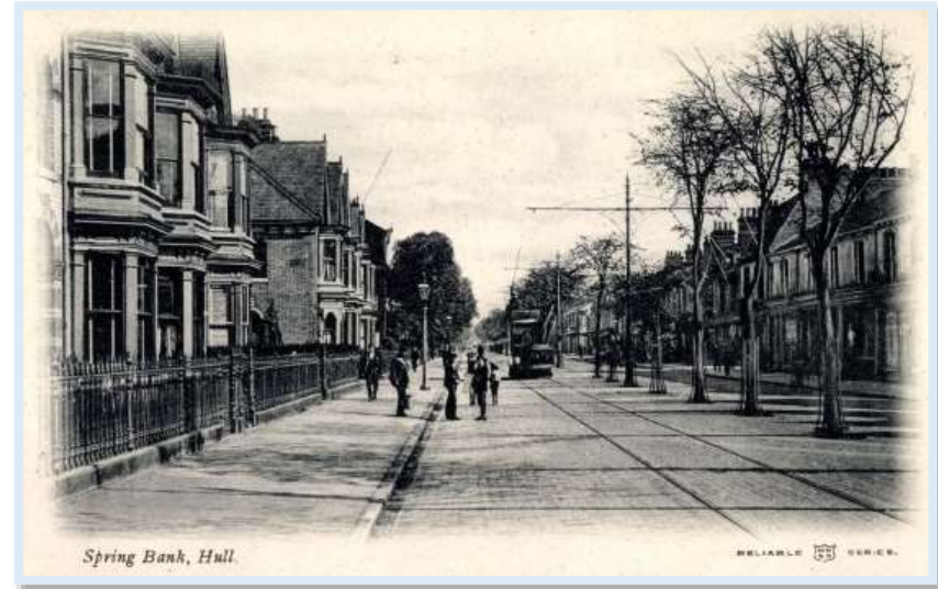
Figure 15 - Historic photograph dating from the late 1800's looking south-east along Spring Bank ( Hull Daily Mail, 2023)
