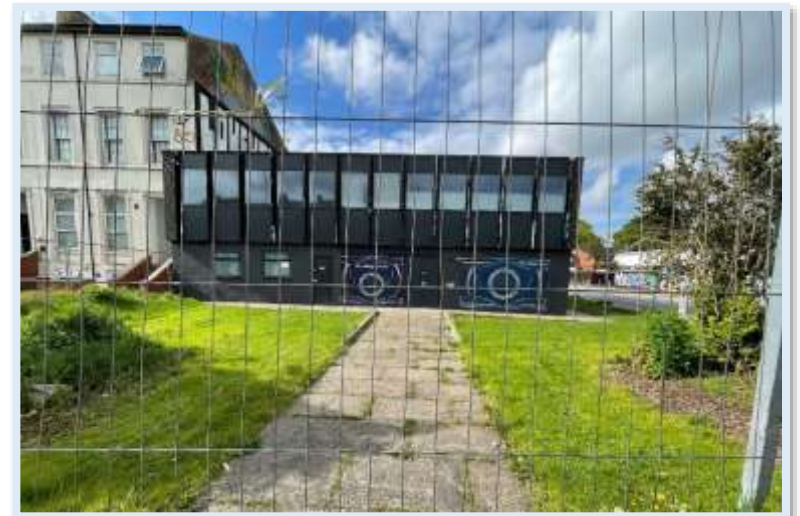
Figure 138 - The frontage of 83 Spring Bank from Spring Bank (Author, 2023)
