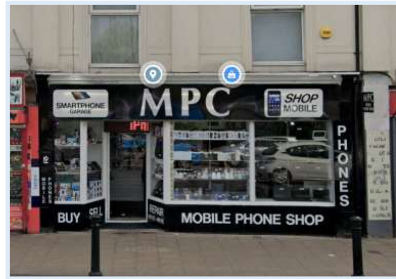
Figure 103 - 19 Spring Bank in 2022 (after designation) with later changes including extensive signage and concealment of the fanlights that has a negative impact on the quality of the shopfront. (google maps, 2022)
