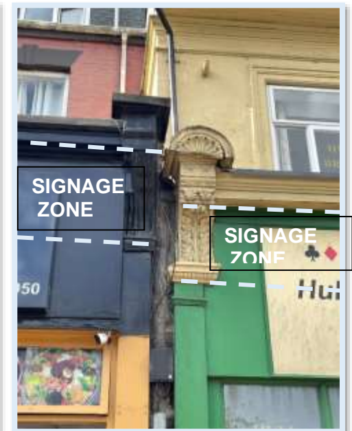
Figure 107 - 115-117 Spring Bank showing how the depth of the signage has increased beyond the original signage zone (Author, 2023)
