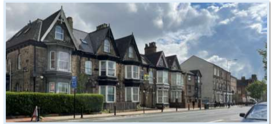
Figure 45 - Photograph of 150 to 168 Spring Bank (north) (Author, 2023)
