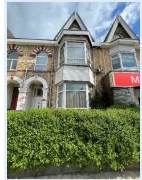
Figure 62 - Photograph towards 174 Spring Bank (north) (Author, 2023)
