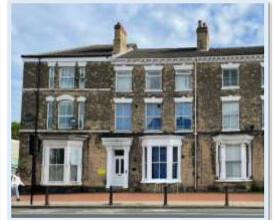
Figure 82 - Pitched roof with limited detail at roof level with the exception of the timber gutter supports. (Author, 2023)
