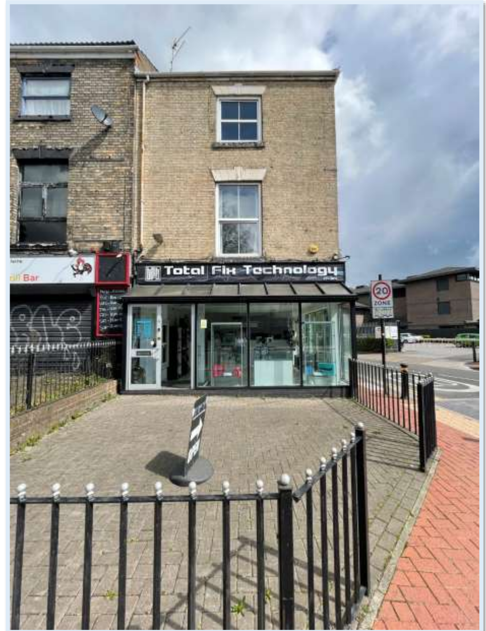
Figure 136 - The Spring Bank frontage to 46 Spring Bank (Author, 2023)
