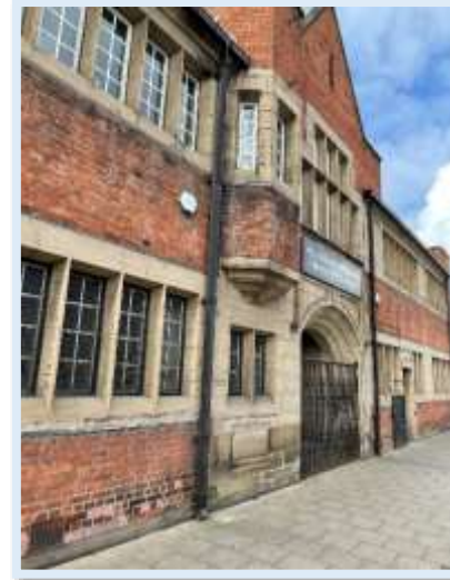
Figure 72 - The use of terracotta brickwork to the Deaf Institute built in the 1920's. (Author, 2023)
