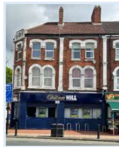
Figure 74 - The use of terracotta brickwork to the Late Victorian buildings towards the west of Spring Bank. (Author, 2023)
