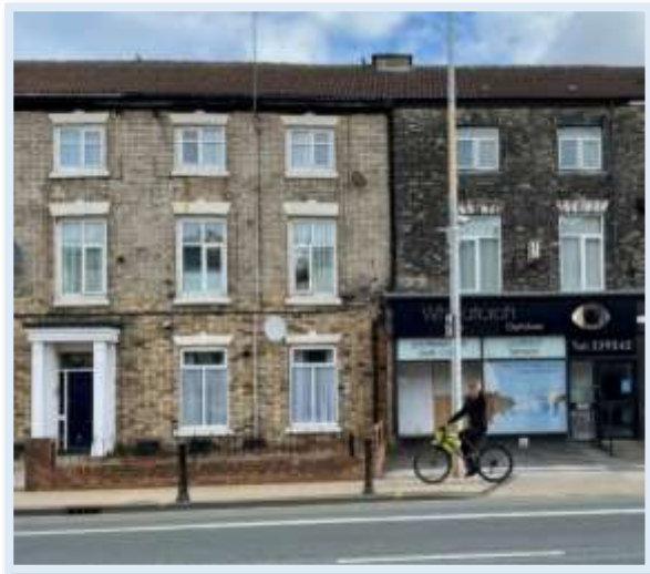
Figure 73 - The use of buff brickwork to the Georgian buildings dating from pre 1830. (Author, 2023)
