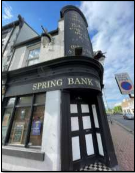
Figure 96 -The original cornice and fascia, shopfrontage at the Spring Bank Tavern (Author, 2023)
