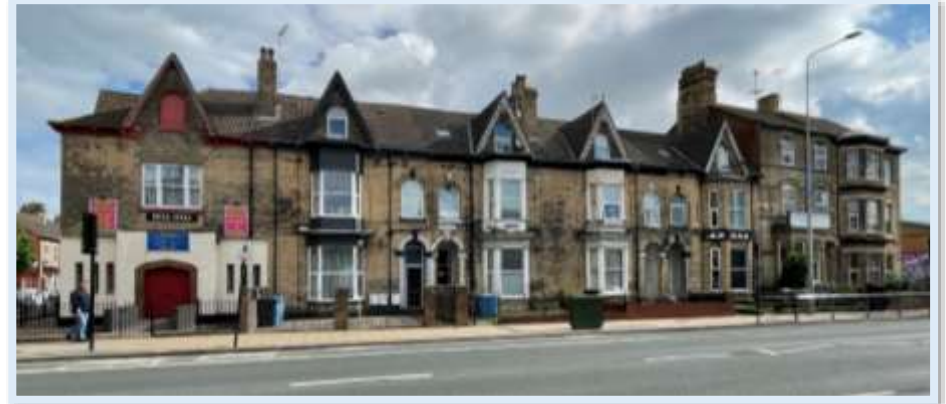
Figure 43 - Photograph of 136 to 148 Spring Bank (north) (Author, 2023)
