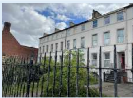
Figure 65 - Photograph of 69-79 Spring Bank showing the low brick wall and piers with iron railings between (Author, 2023)
