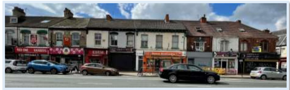
Figure 48 - Photograph towards 147-167 Spring Bank (south) (Author, 2023)
