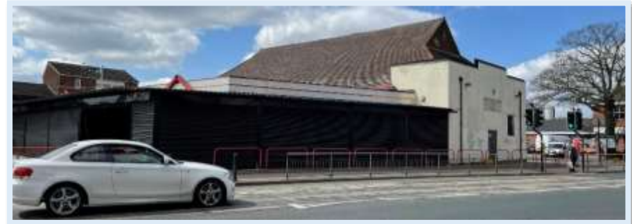
Figure 132 - Retail unit that extended the former Church Hall to St Jude's Church creates a negative frontage and lacks quality (Author, 2023)
