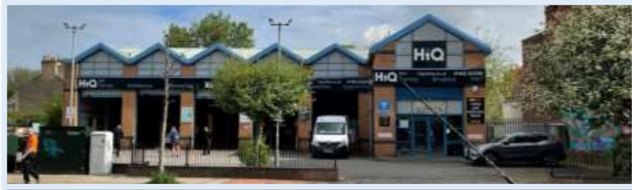
Figure 57 - Photograph towards 124-134 Spring Bank (north) (Author, 2023)
