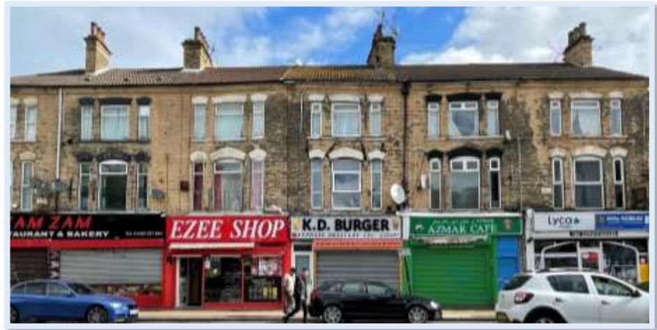
Figure 58 - Photograph towards 100-112 Spring Bank (north) (Author, 2023)
