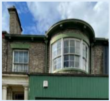
Figure 89 - Original timber sliding sash windows retained (Author, 2023)
