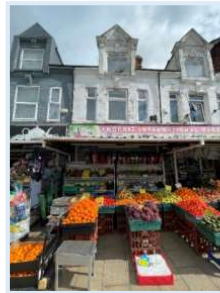
Figure 61 - Photograph towards 198 Spring Bank (north) (Author, 2023)
