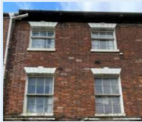
Figure 90 - Original timber sliding sash windows retained (Author, 2023)
