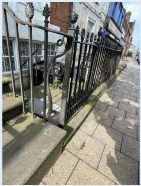
Figure 88 - Decorative wrought iron railings with serpent supports (referencing the Zoological Gardens) providing a high quality boundary treatment to 53-55 Spring Bank (south) (Author, 2023)
