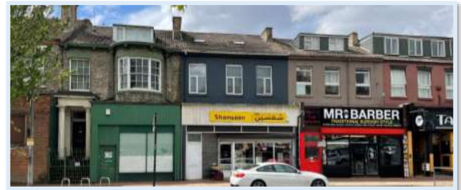
Figure 126 - 109-113 Spring Bank showing how later addition shopfronts and uPVC windows have reduced the quality (Author, 2023)
