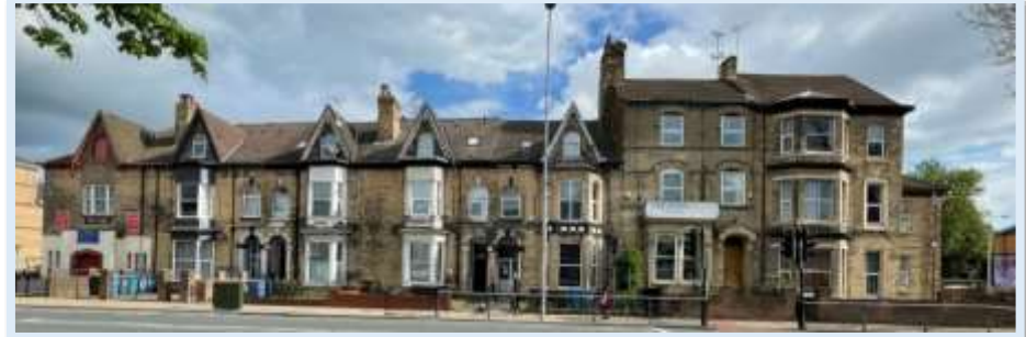
Figure 55 - Photograph towards 136-148 Spring Bank (north) (Author, 2023)
