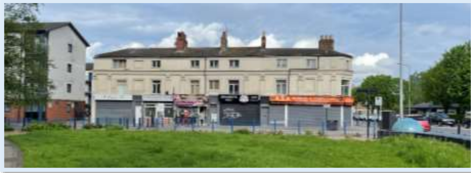
Figure 150 - View towards Spring Bank from Ferensway looking across Spring Street (Author, 2023)
