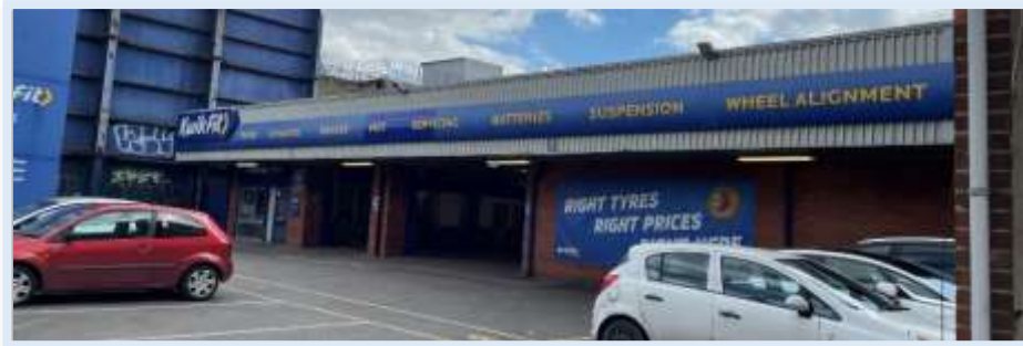
Figure 130 - Kwik Fit garage built on the site of a former Chapel (Author, 2023)
