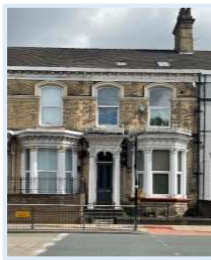
Figure 75 - The use of buff brickwork to the Late Victorian buildings towards the west of Spring Bank. (Author, 2023)
