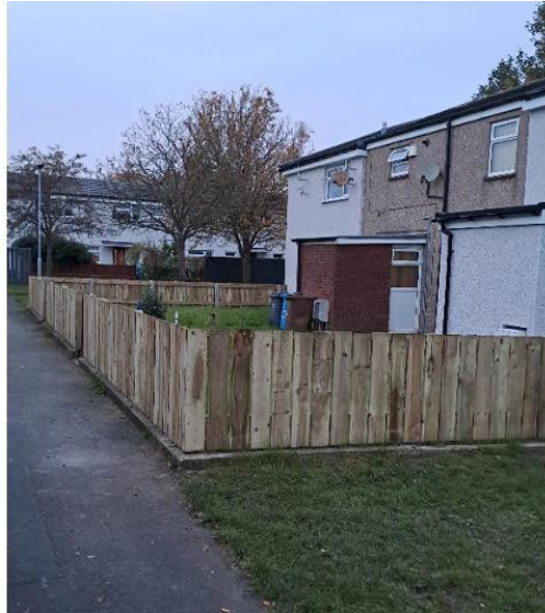
Wenlock st gates and fencing
