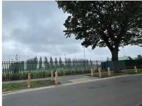
Bollards on Inglemire lane
