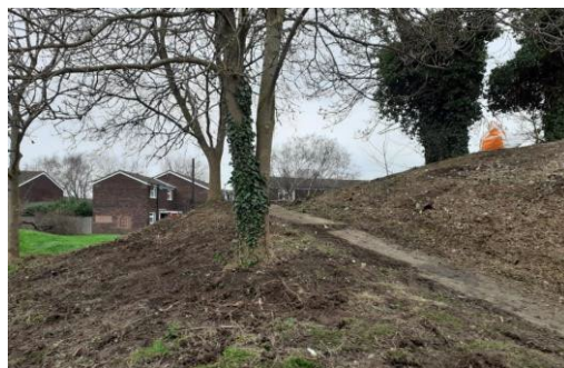
Vane st park mound clearing
