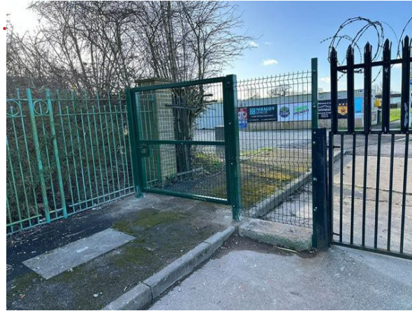
New gate at entrance to Kingswood United Football Club
