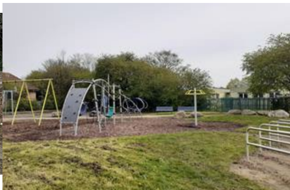
Liddell st park refurbishment
