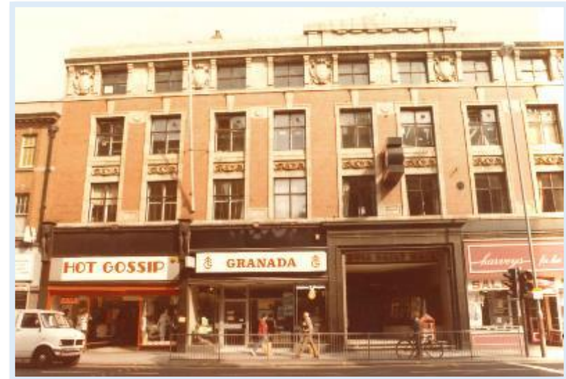
Figure 3 Demolished Hull Daily Mail Buildings, Jameson Street c.1990
