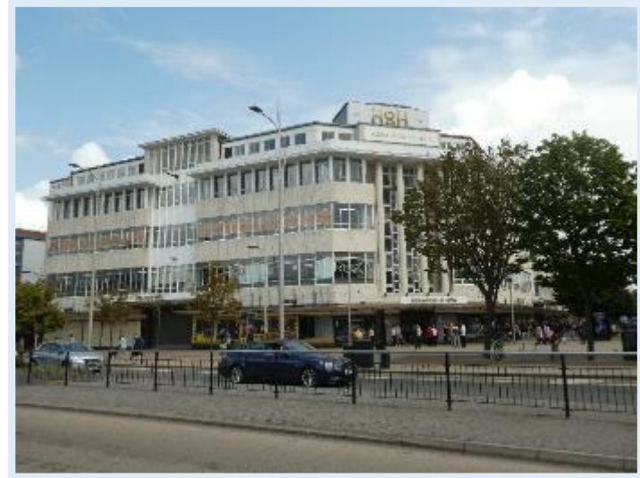
Figure 99 View from Paragon Station
