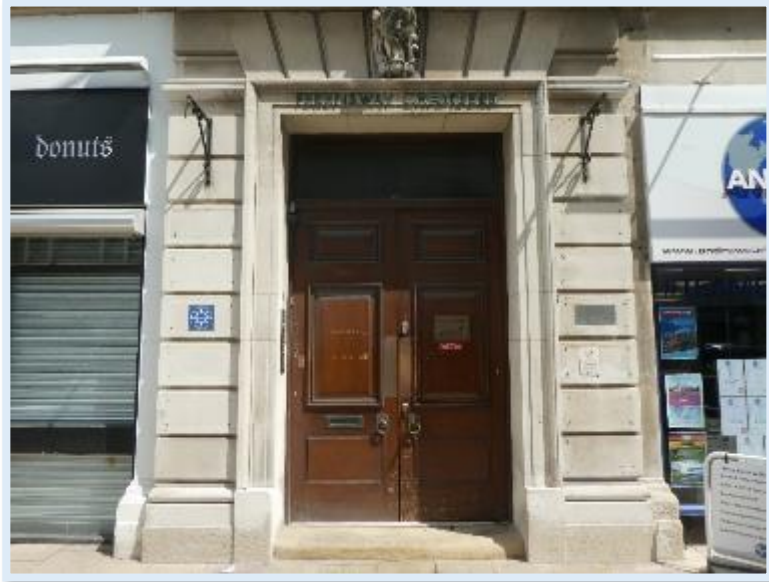
Figure 66 Original Door at Ferensway Chambers
