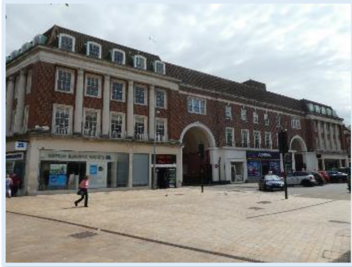
Figure 62 Uniform Appearance to windows at Queen's Buildings
