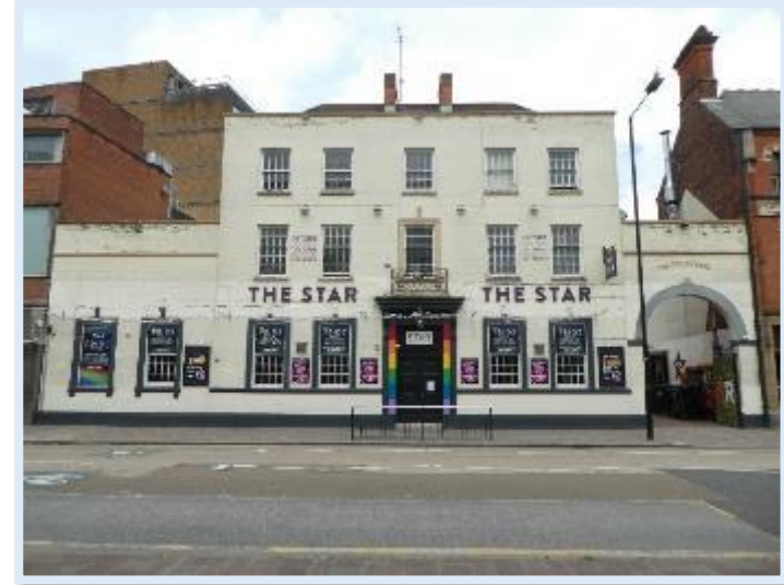
Figure 60 - Georgian Revival Inn on Carr Lane
