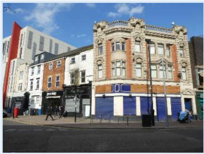
Figure 83 Positive Buildings at Story Street and King Edward Street
