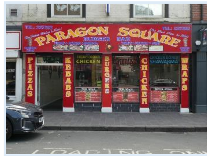
Figure 56 'Cluttered' Shop front at 14 Paragon Square
