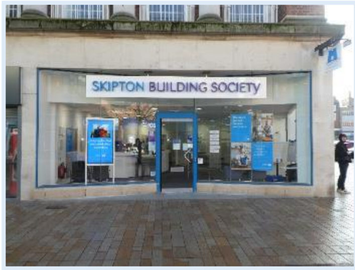
Figure 44 Good quality shop front at Queen's House
