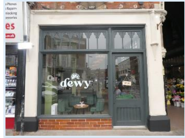
Figure 41 Grade II Paragon Arcade contains reproduction and replacement Gothic Joinery
