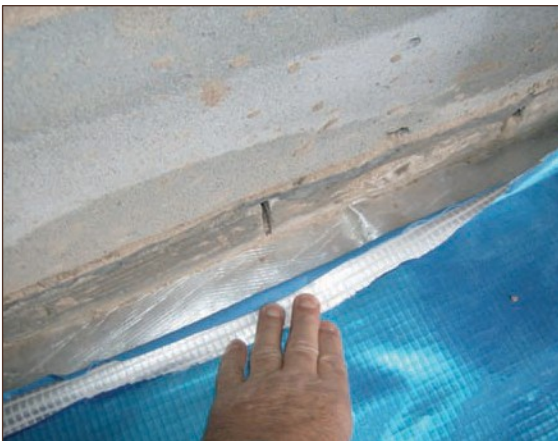
Figure A4.77 Small lap and no single sided tape used to achieve secondary seal (courtesy Smith Grant)
