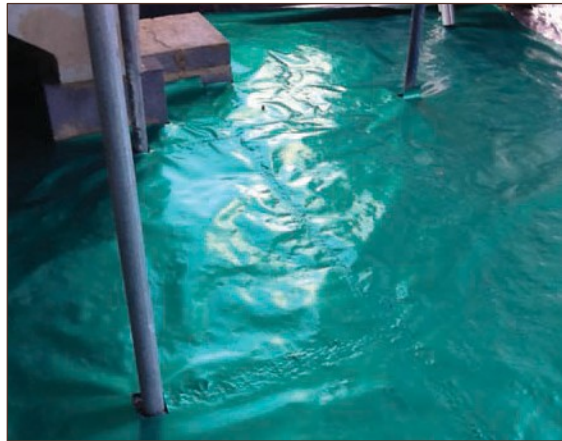
Figure A4.52 Gas membrane cut by scaffolders and bricklayers after installation (courtesy MEC Environmental Ltd)
