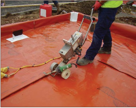
Figure A4.31 Extrusion welding (courtesy PAGeotechnical Ltd)
