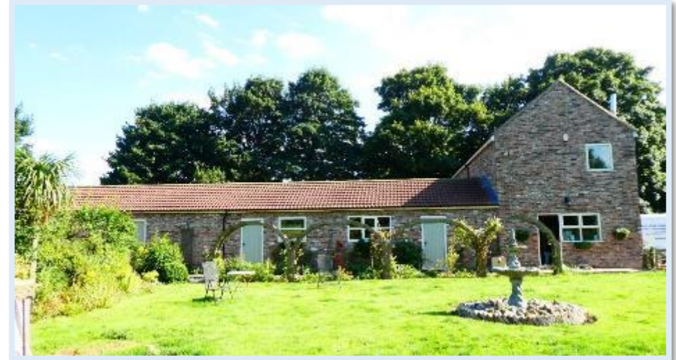
Figure 19 Rural outbuildings of Brickyard Cottage
