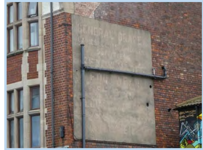
Figure 98 Gable wall of No.142 – 'General Draper'
