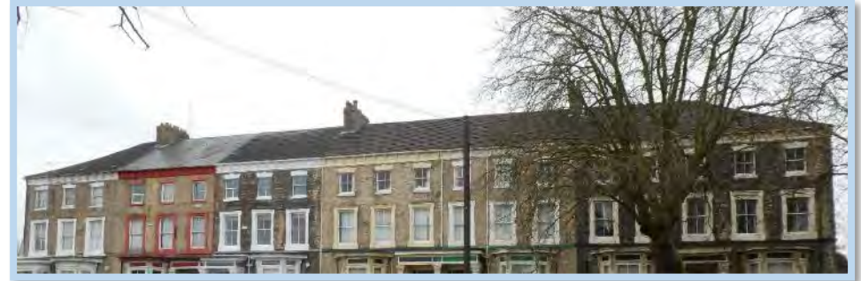
Figure 127 Nos 72-84 (Grade II) - Mid-19th century roof without dormers. Only one section retains traditional slates.
