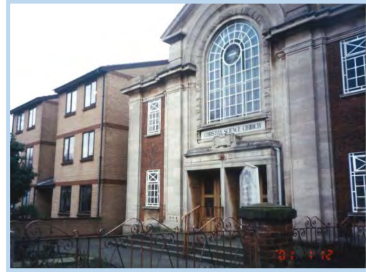
Figure 111 No.383 before extension.
