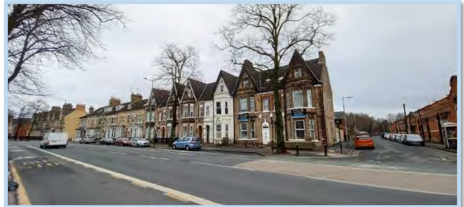
Figure 163 Positive quality terraced housing in Zone 3
