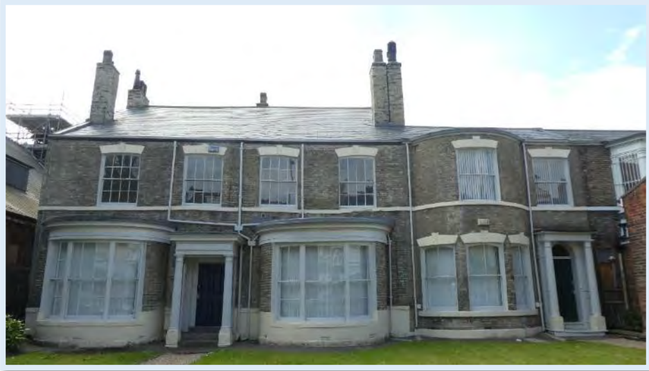
Figure 42 Nos.53 & 55 - 'York Terrace'
