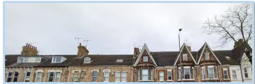
Figure 128 A negative quality roof scape - mixed use of modern dormers, roof lights and materials.
