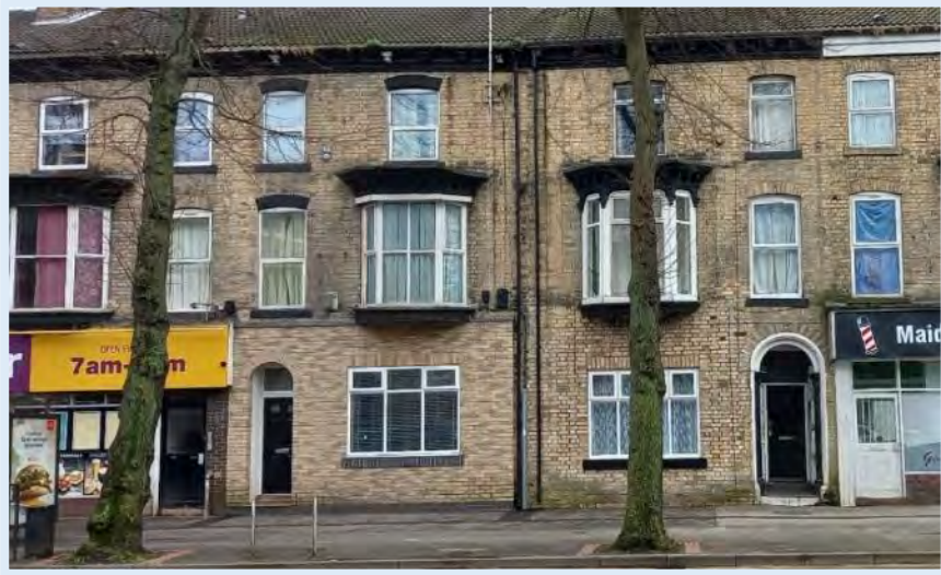
Figure 207 Nos. 213 & 314 Ground floor re-instatements without architectural decoration.
