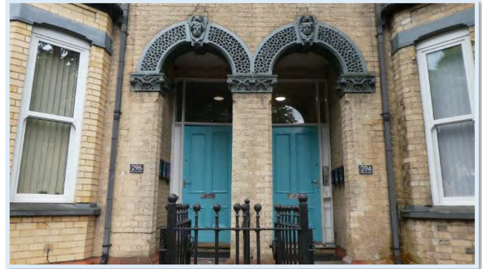
Figure 125 Nos.294-296 -Late 19th century 4 panel doors, in pairs.
