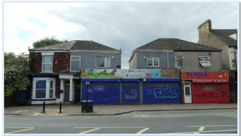
Figure 88 Nos.201-207 - Poor quality shop front additions.
