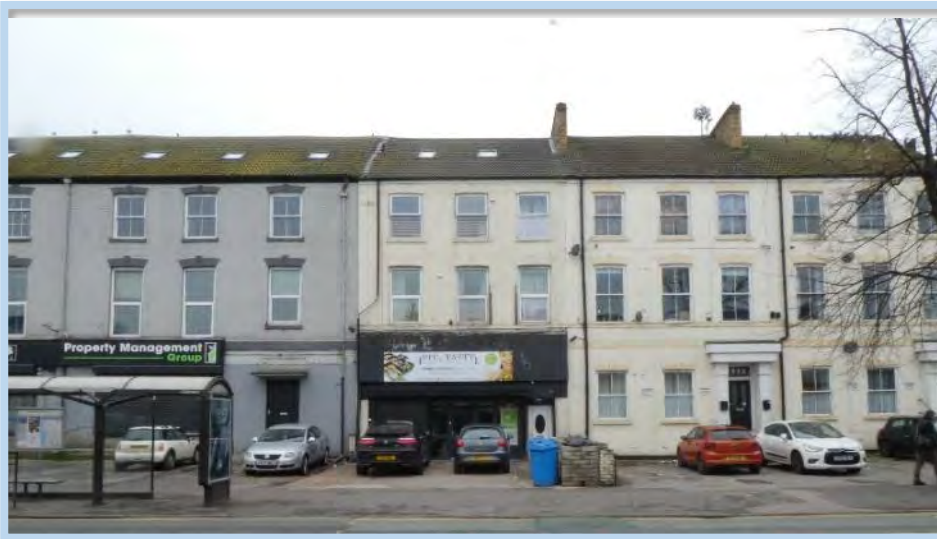
Figure 114 - No.113 showing loss of uniform appearance to terrace.
