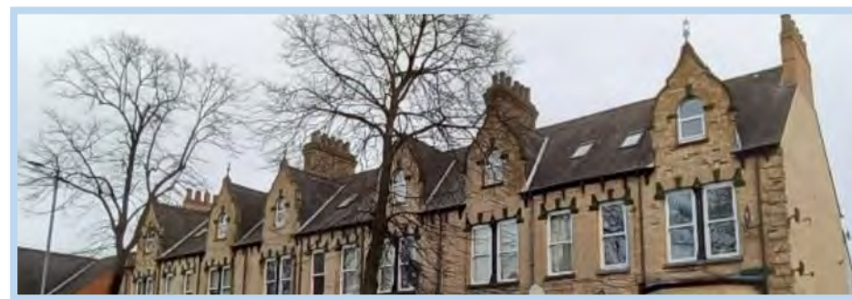
Figure 135 Nos. 286-96 (Local Listed) - Shaped gables & traditional materials..
