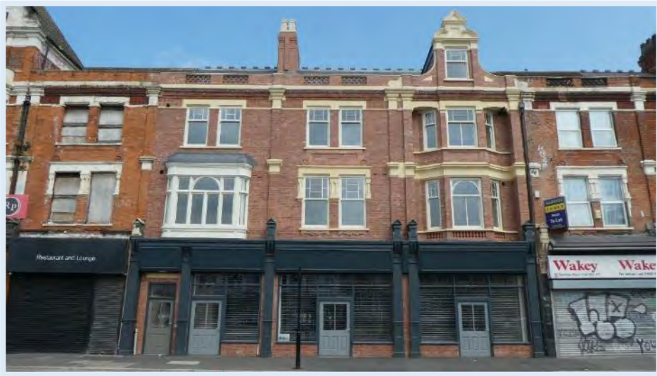
Figure 9 Brunswick House re-built and new shop front.
