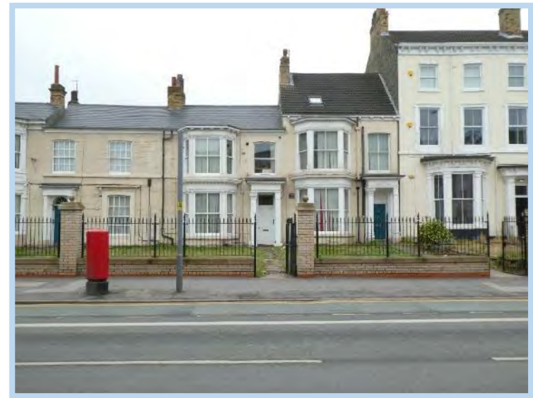
Figure 153 Nos.85-87 forms a positive grouping of early 19th century buildings, with traditional joinery detail. Boundaries restored THS.
