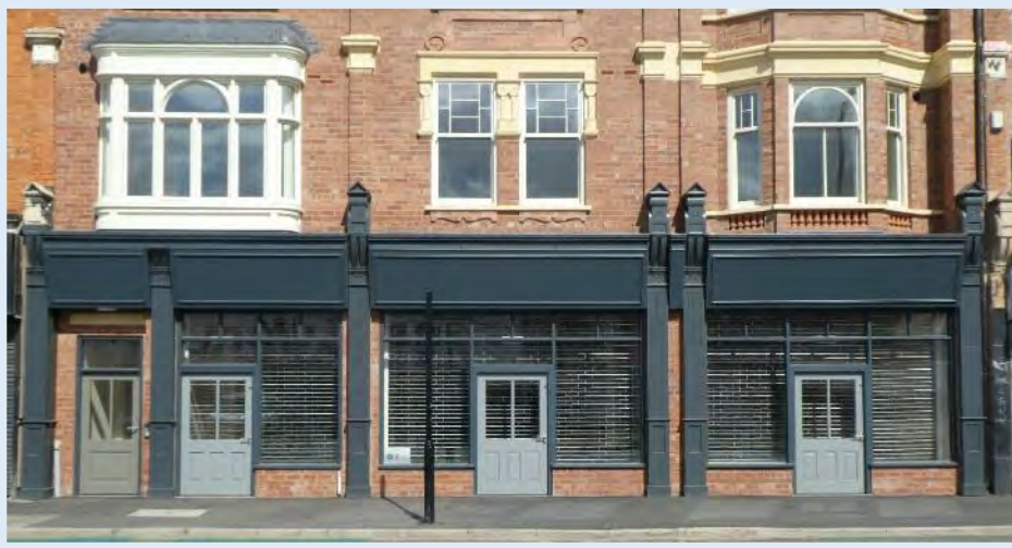
Figure 74 No.52-52a - THS shop front restoration, which incorporates the historic columns on the Brunswick Arcade.
