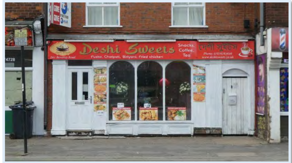
Figure 76 No. 241 - A positive quality c.1990s arched shop window.
