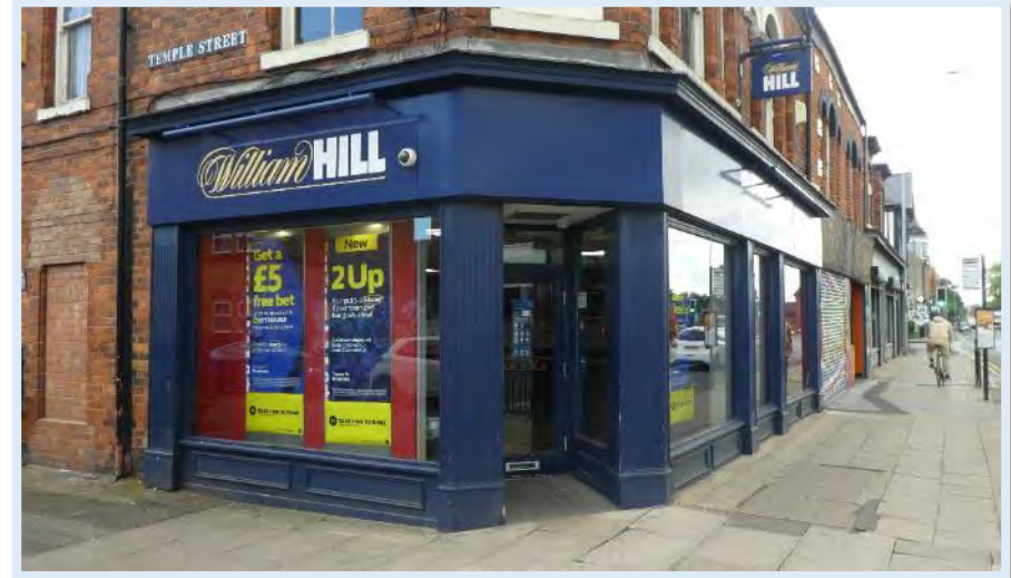
Figure 71 No.214 - good quality late 20th century shop front.
