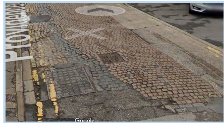
Figure 194 Historic setts in Providence Row (Google images)
