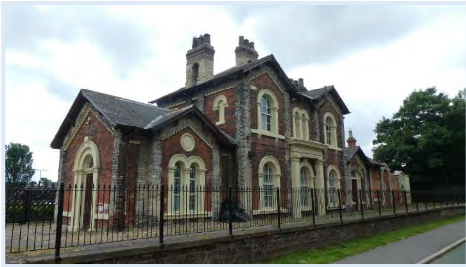
Figure 108 Stepney Station House (Grade II) & platforms, with restored railings (THS)
