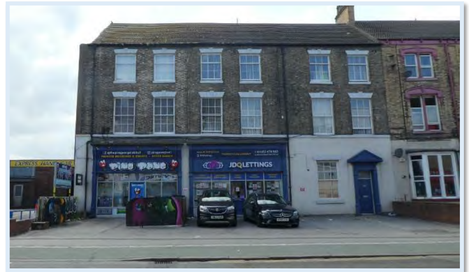
Figure 11 - Nos. 129-31 after restoration.
