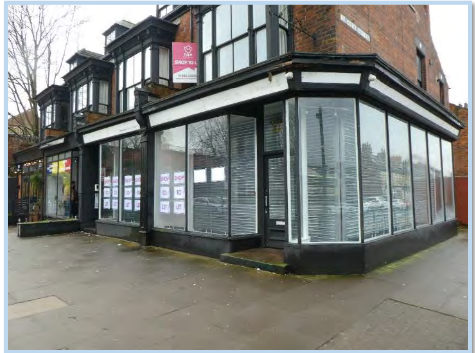
Figure 66 No. 323-341 - A key shop front within the Conservation Area, constructed between 1889/9 and 1906.
