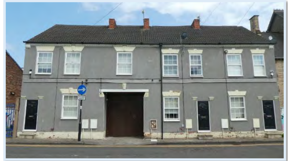
Figure 33 - Recent enhancements along Grosvenor Street
