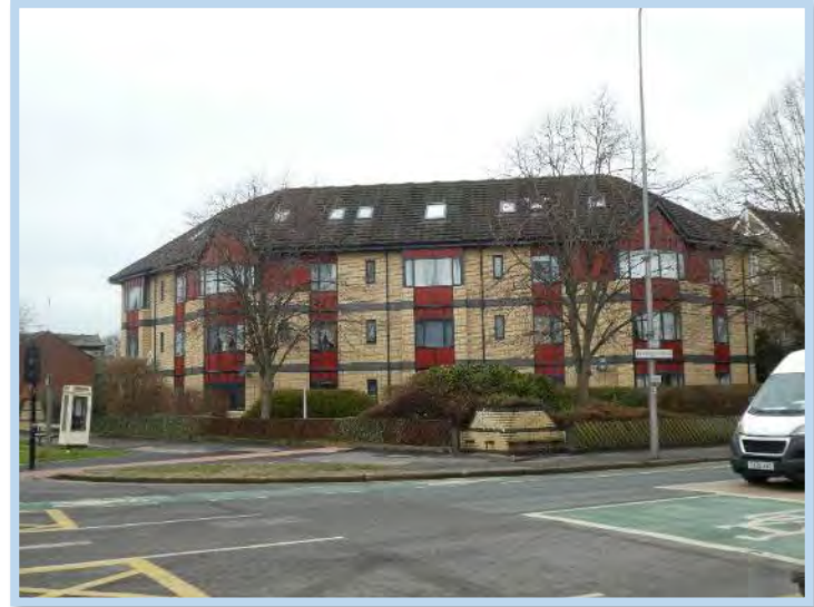
Figure 175 Prominent modern development of junction of Queen's Road
