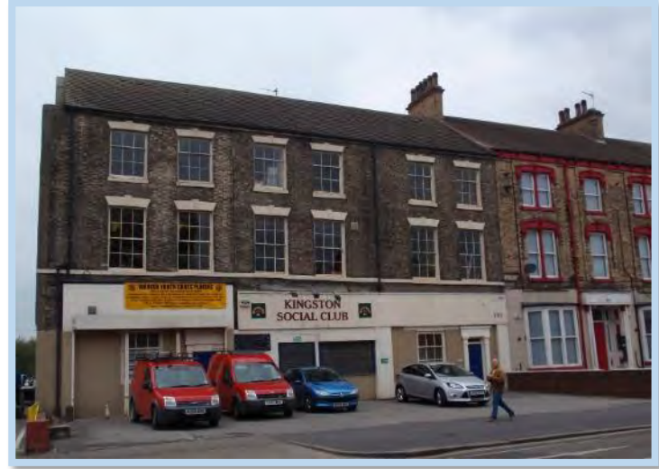
Figure 10 - Nos. 129-31 before restoration.
