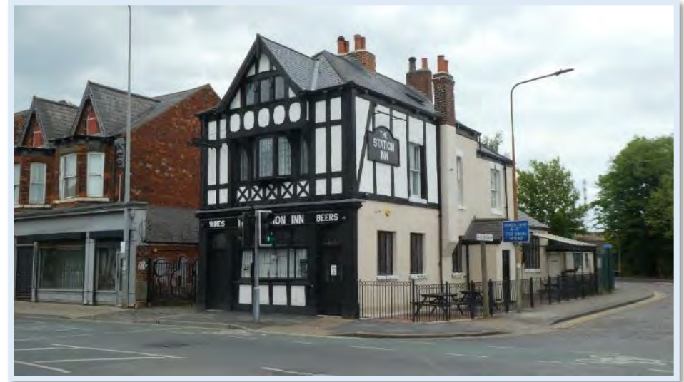
Figure 102 0 Station House (Local Listed) - Restored THS.
