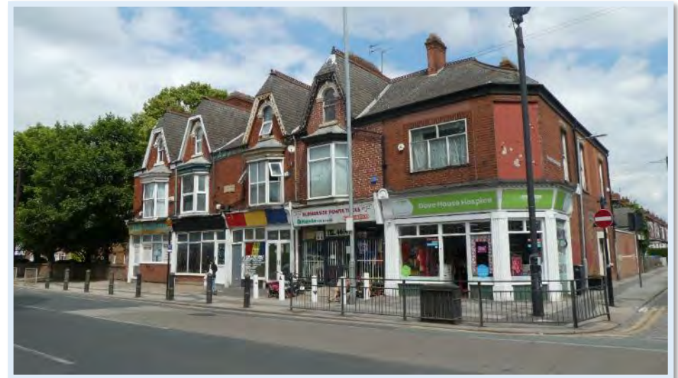
Figure 1 – Nos.433-40 Typical positive buildings of Zone 4.
