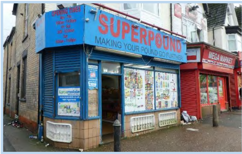
Figure 86 Nos. 414 and 416 - The prior retains a historic stall riser, but the shop fronts are of a poor-quality (showing condition before alteration in c.June 2024).
