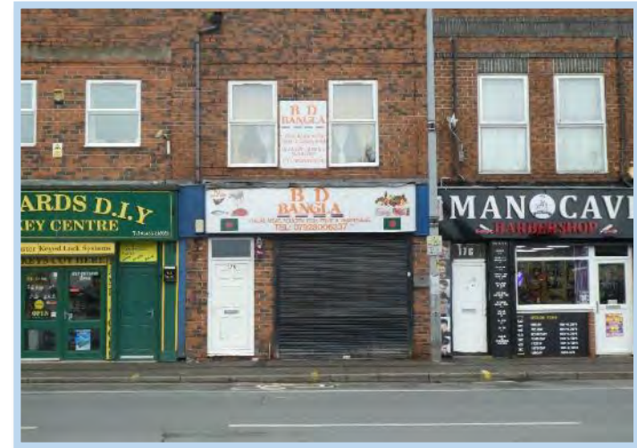
Figure 169 No positive feature retained at No.178
