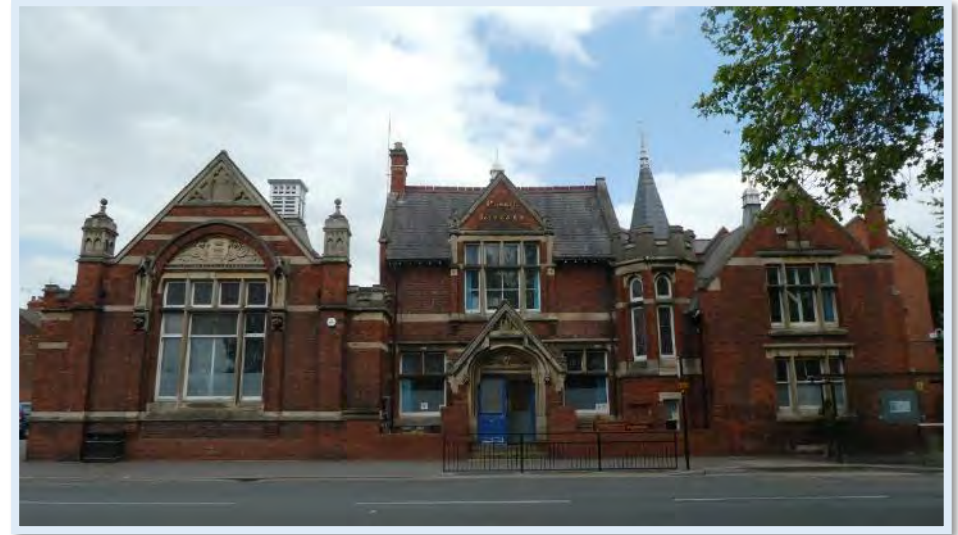
Figure 100 Grade II Northern Branch Library
