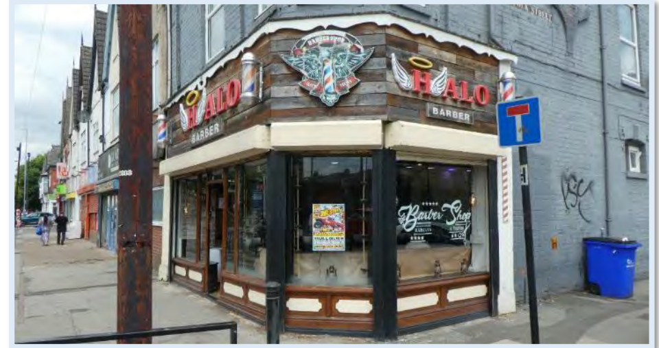
Figure 91 No.414 - Positive element of a timber shop front but with poor quality advertisements.
