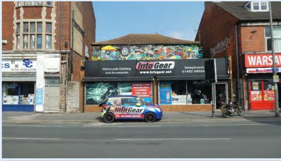
Figure 93 Poor quality ground floor frontages at No.140
