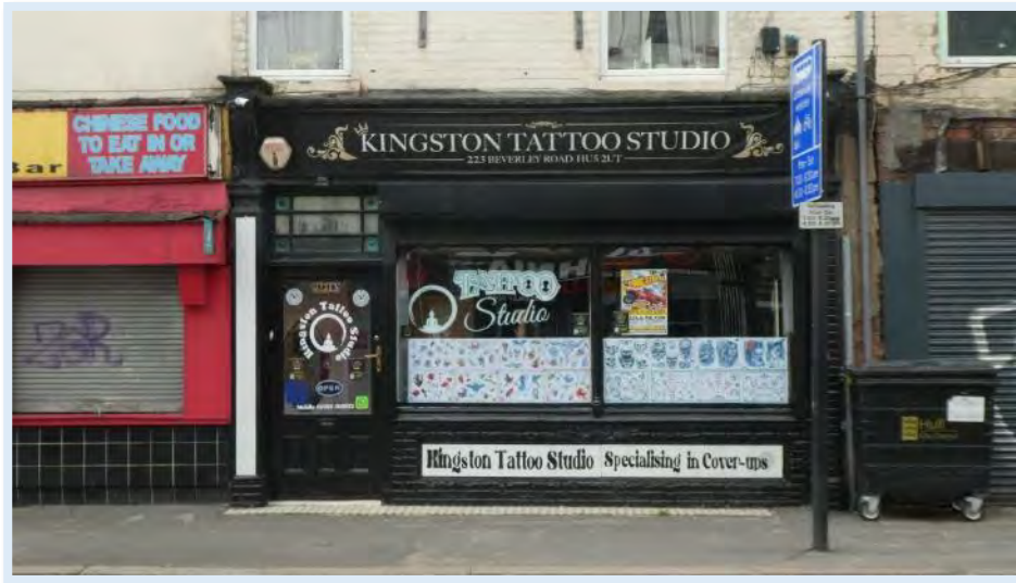
Figure 68 - No.223 - Surviving late 19th century shop front.
