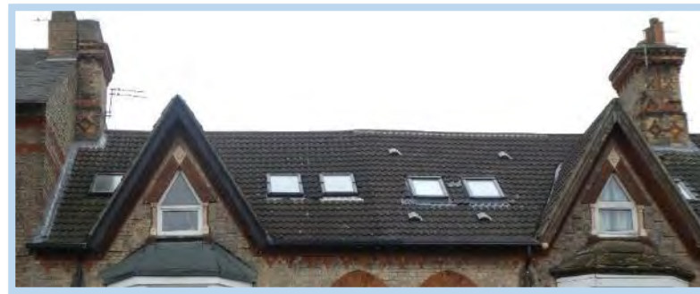
Figure 133 Cluttered roof profile at Nos.96-8
