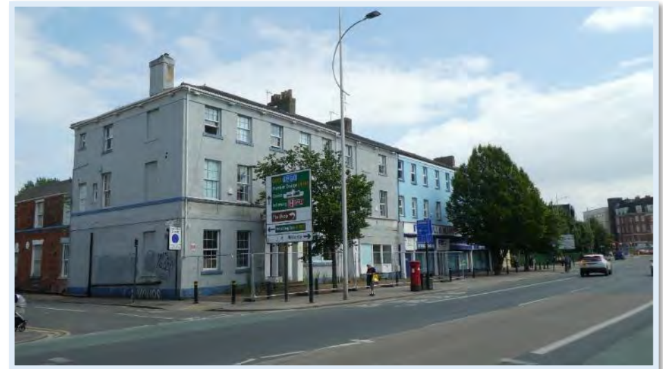
Figure 15 Nos.32-43 Beverley Road
