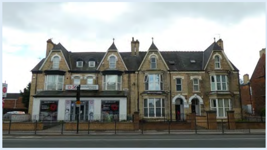
Figure 113 - Loss of domestic frontage at No.407-409.
