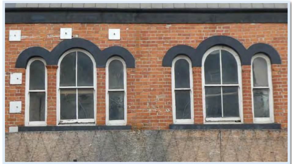
Figure 120 No.214 - Venetian windows, with 2/2 sliding sashes with historic glass.
