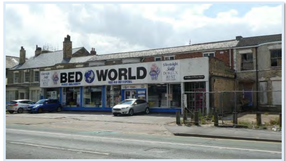
Figure 65 Extension added to Nos.57-59 in c. 1900
