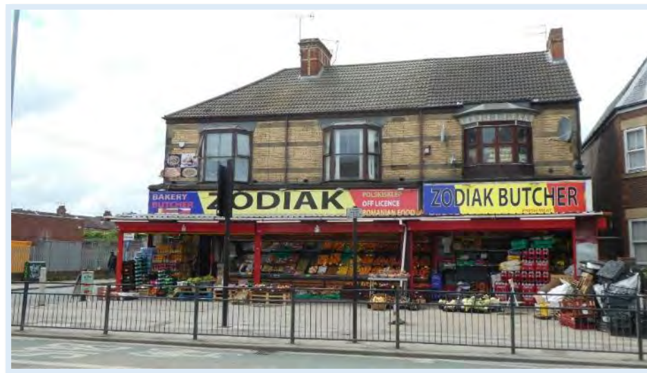
Figure 90 Canopy at 359 Beverley Road (Pending Enforcement at time of survey)
