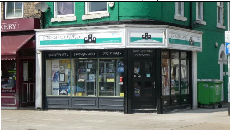
Panelled stallrisers, timber fascia.
