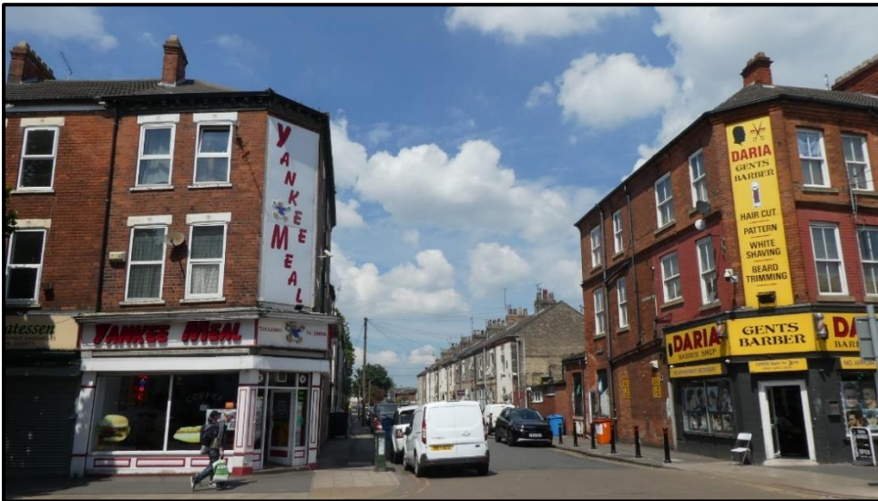
Figure 8. Building corners used as advertising panels.
