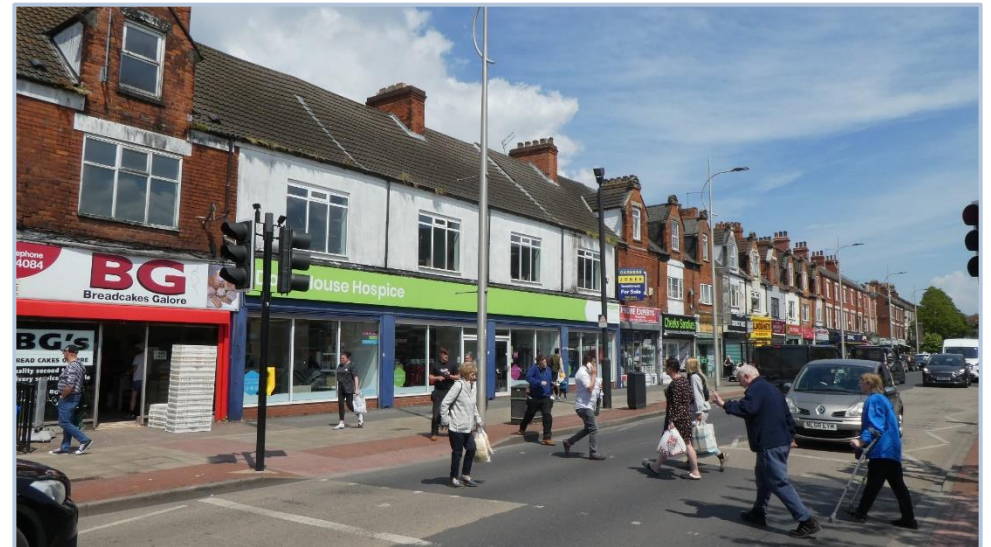
Figure 9. Evidence of dormers on 360-390 Hessle Road, now lost. 2008 vs 2024. Source: Google Street View; Stephen Walker.
